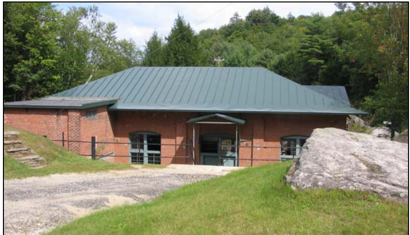
Photograph 3: New standing seam metal roof on Cavendish generating station, September 10, 2009.
