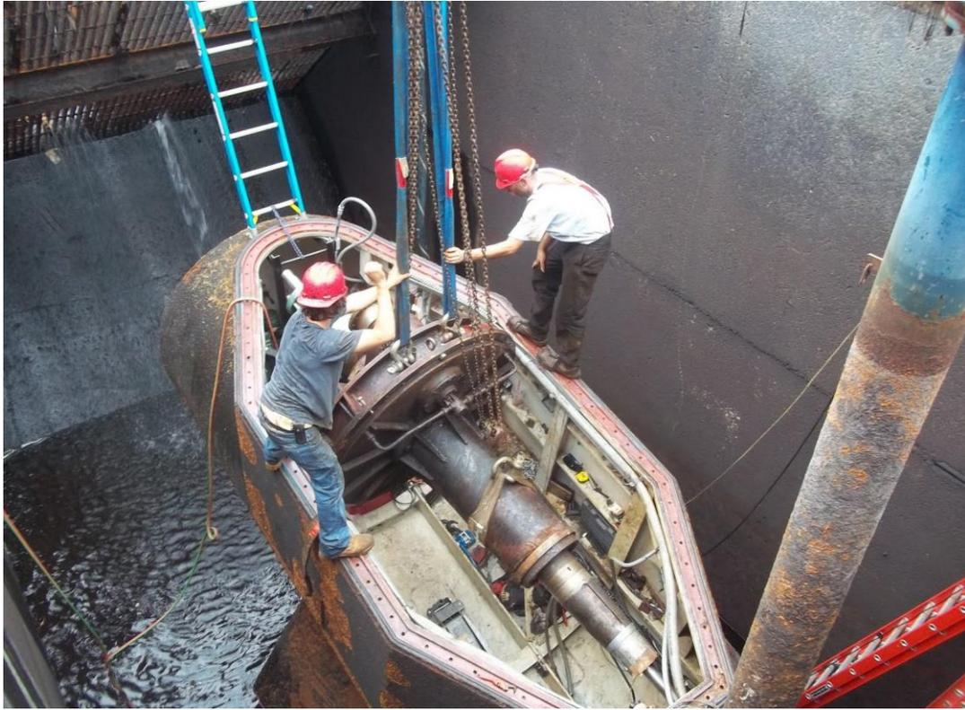
**Installing the refurbished gearbox after 45 days at Electro Mechanics in Springfield, MA**
