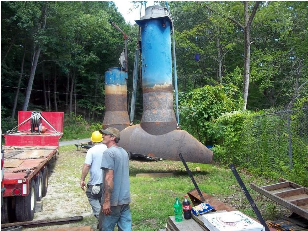
**The top of the bulb is the last component for the crane to lift back to the flume location in the river**
