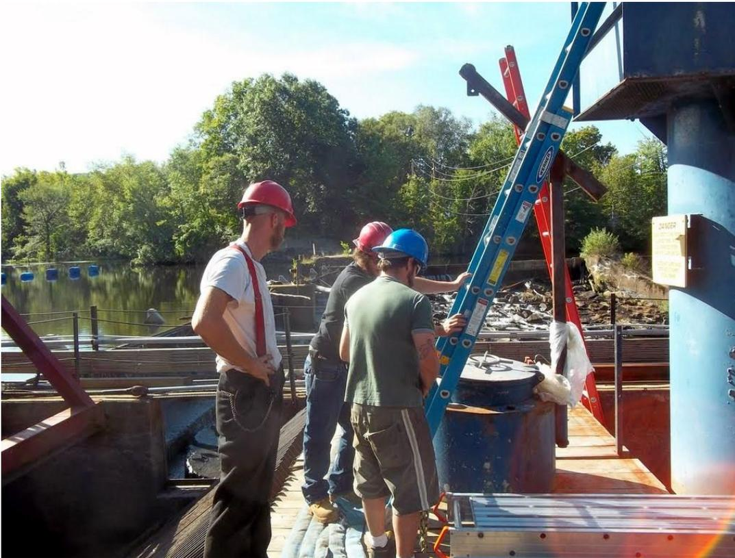
**Preparing to remove the bulb top so the gearbox can be extracted from the nose cone.**
