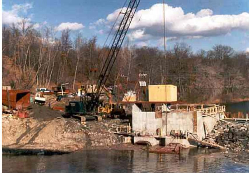
**Collins Hydro project: setting the draft-tubes during construction in 1984**
