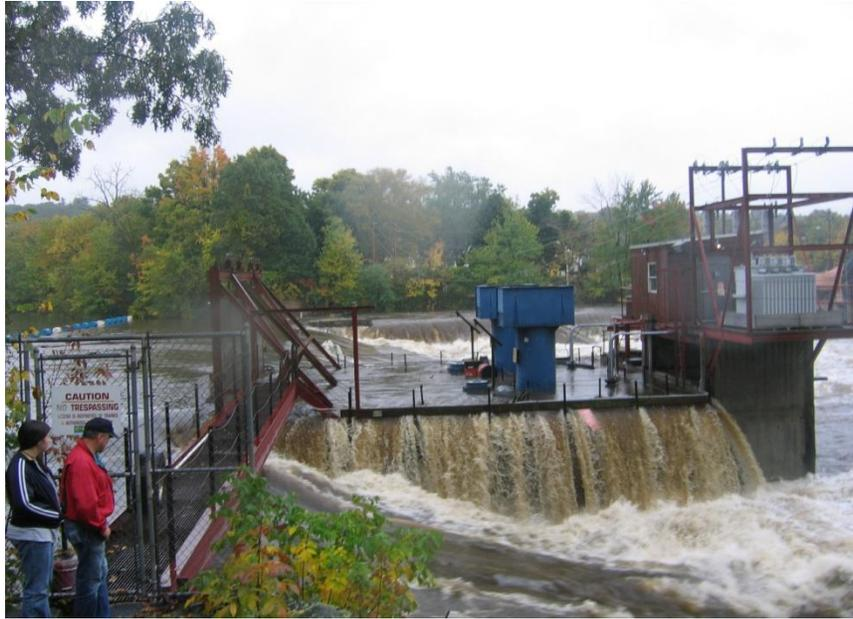
**In flood Collins bulb turbines as safe and continue to generate, flashboards are lowered**
