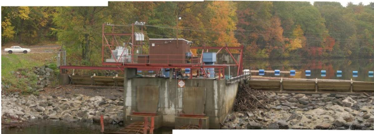
**The hydraulic operators lift the hinged flashboards to 4 feet, but could be replaced with inflated runner crest gates**
