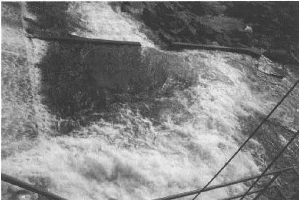
Photo No. 8 – View of the plunge pool for the downstream fish passage facility.
