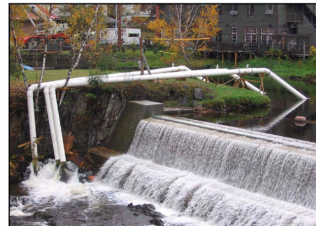
Location 5: Waterflow diversion pipes required by VT ANR during dam construction, looking north in left image and looking southwest in right image. October 10, 2009.
