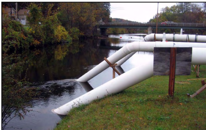
Location 5: Waterflow diversion pipes required by VT ANR during dam construction, looking north in left image and looking southwest in right image. October 10, 2009.
