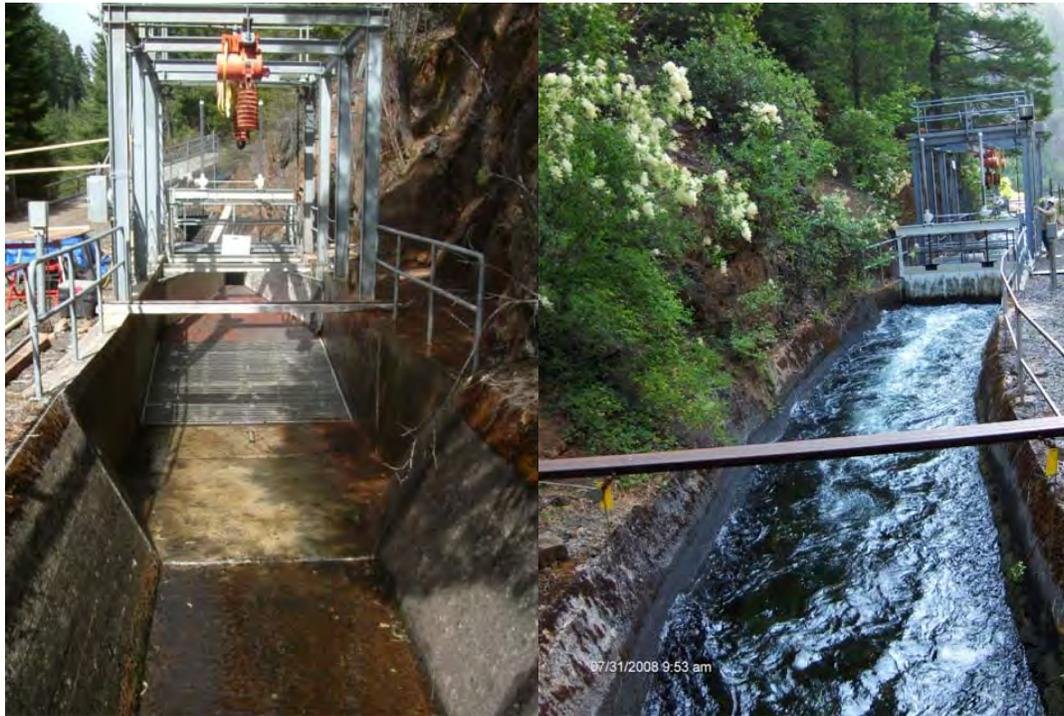
Prospect No. 3 fish screen and downstream fish bypass facility. Photo on left is a view looking downstream along the dewatered canal. The right photo is a view looking upstream with the facility in operation.
