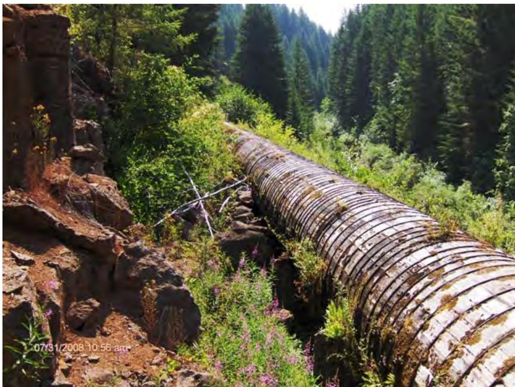
Example of a woodstave pipe section on the Prospect No.3 water conveyance system.
