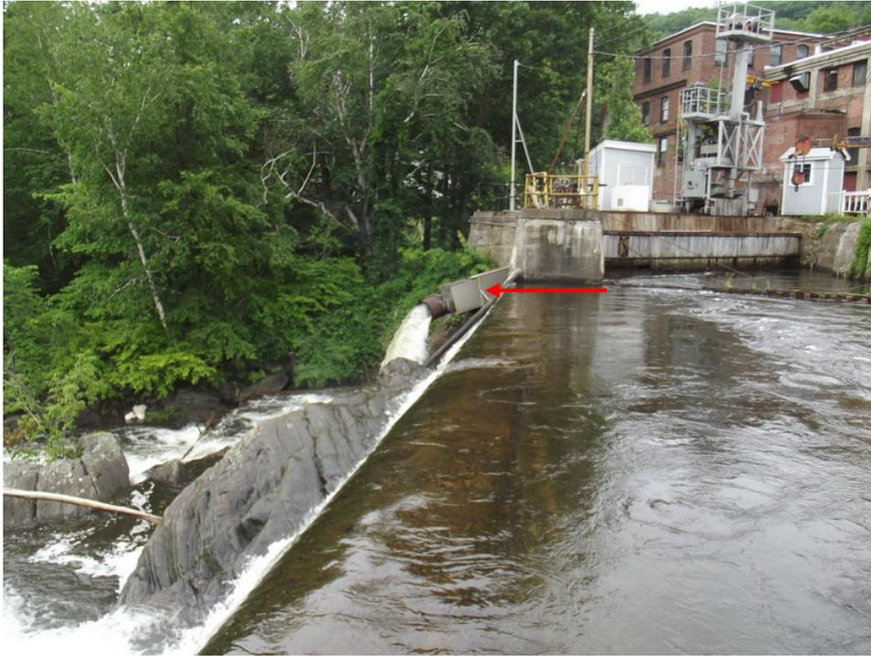
Photograph 5 - View looking at intake and downstream fish passage discharge pipe (arrow).
