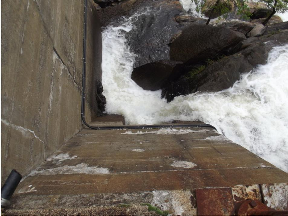
**Photograph 3 - View of minimum flow release through low level gate at the north channel dam.**
