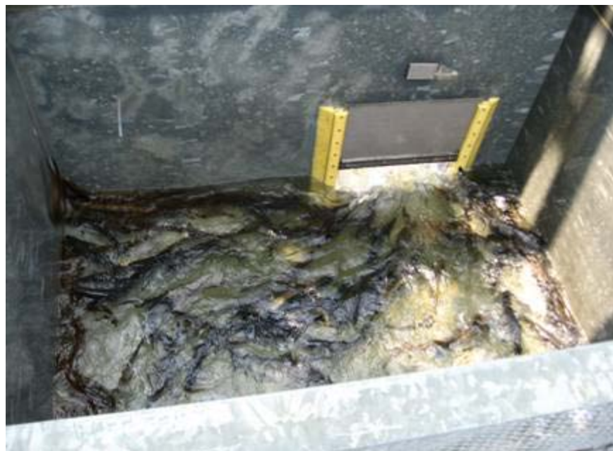
Figure 1-3. Holyoke fish lift. An image of a fish lift hopper near the end of the dump. The perspective is similar to that of observers monitoring fullness.
