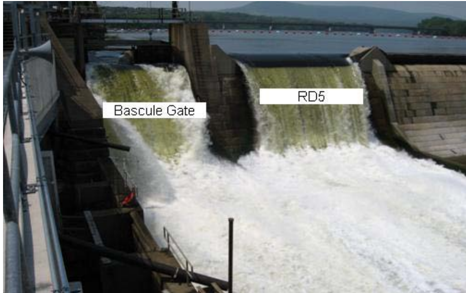
Figure 1-1. Holyoke Dam, Bascule Gate with Alden Weir and Rubber Dam section #5 (RD5). Rubber Dam section #4 is visible in the closed position to the right of RD5.
