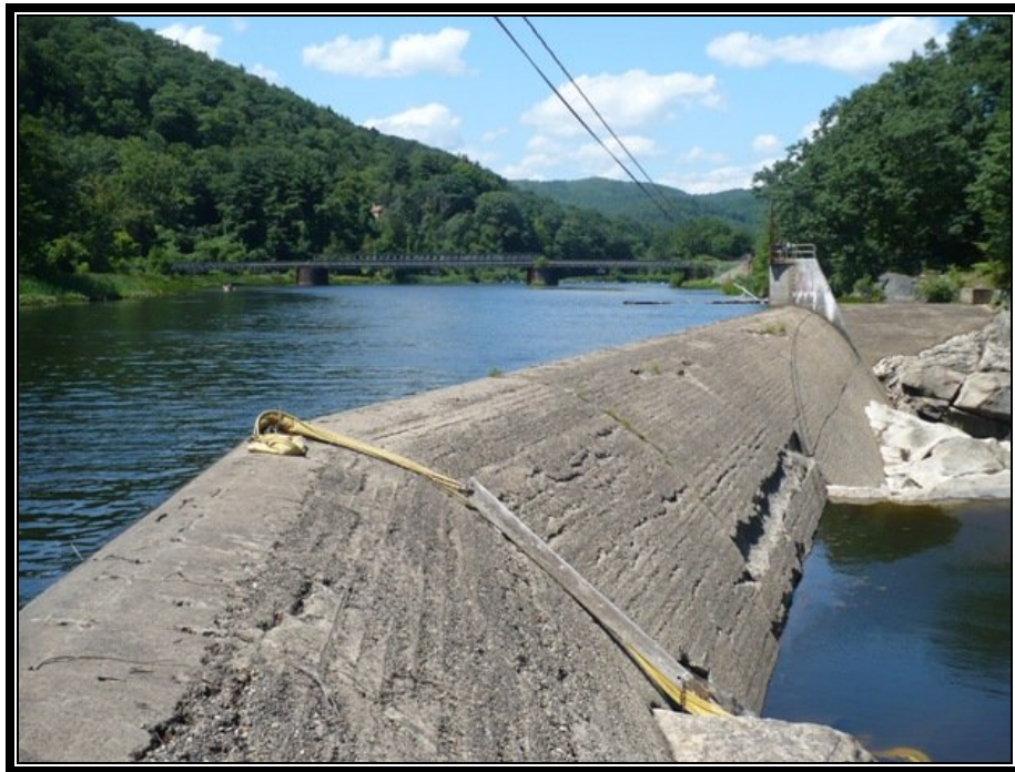
Photo No. 4 – South Dam looking north toward south from the rock outcropping in the Westfield River. Note the gouges at the dam surface, the Licensee proposed to repair the remaining gouges at a later date.
