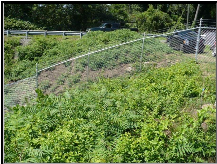
Photo No. 14 - Crest of the earth dike looking longitude toward the south. Note the overgrown vegetation (not on photo location map). Note the licensee was requested to remove the vegetation.
