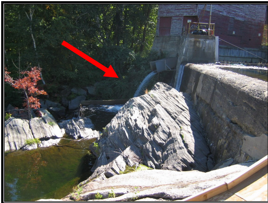
Photo No. 18 – View of the fish passage chute. Note fish passage was not in operation. However, the flow releases (at red arrow) was satisfying the project minimum requirements.
