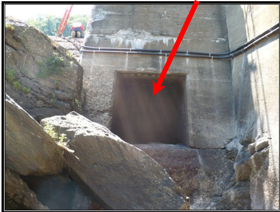
Photo No. 20 - View of the flow releases (at red arrow) from opening of the north side mud gate to satisfy the project minimum requirements.
