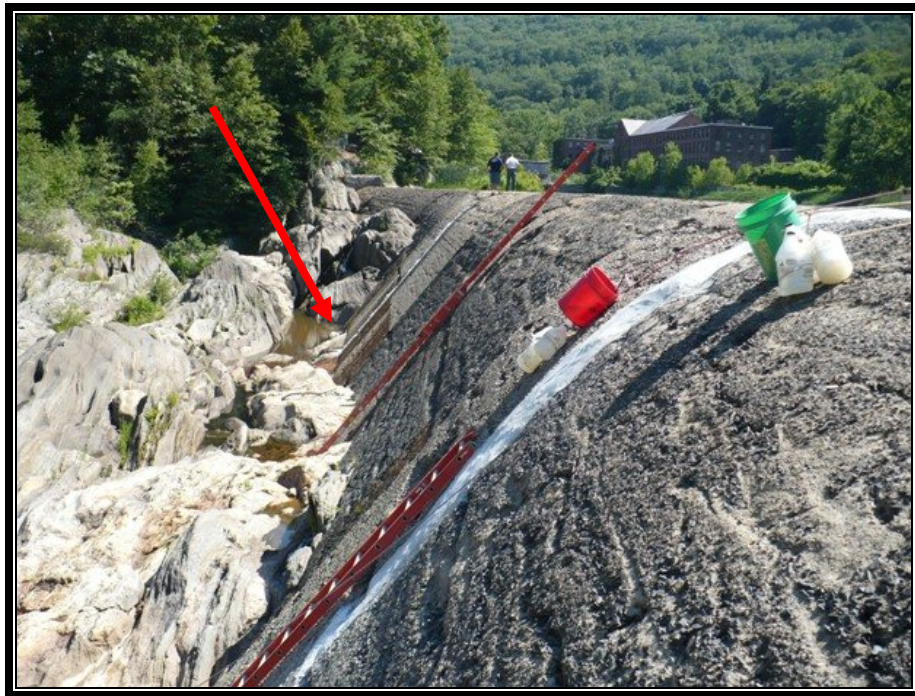
Photo No. 3 – North Dam looking toward south from the left abutment gate structure. Note the repairs being made to the dam surface.
