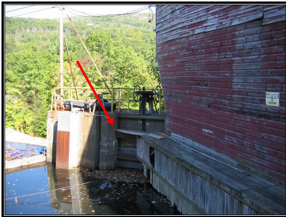
Photo No. 6 – View of the sluice gate adjacent to the intake Structure.
