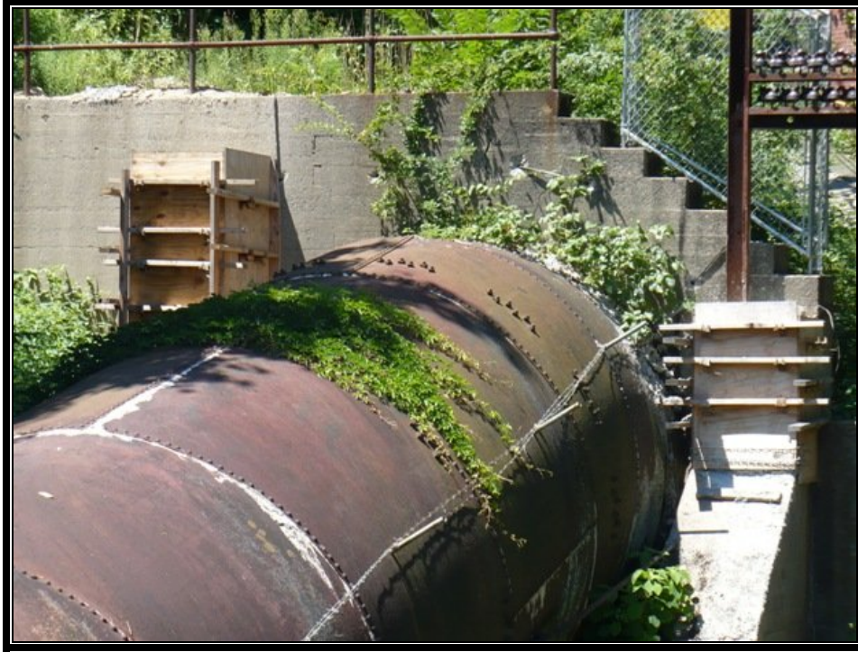
Photo No. 9 – Close view of repairs made to concrete piers supporting penstock.
