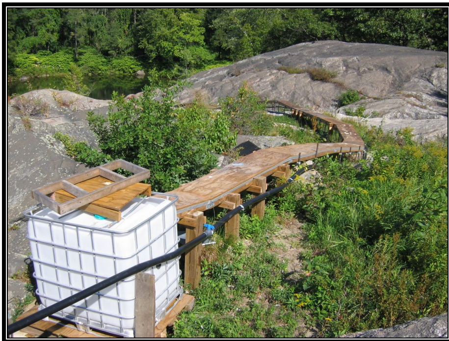
Photo No. 21 – View of one of the three eelways that was constructed for monitoring of the eelway effectiveness studies.
