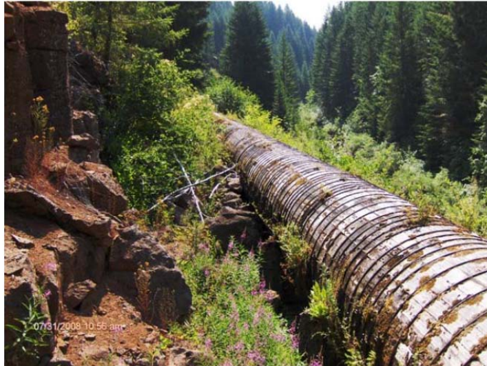
Section of woodstave water conveyance system.
