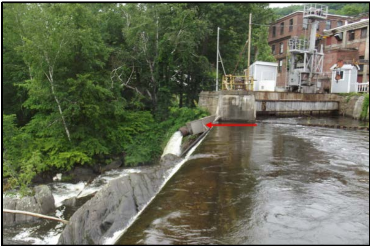
PHOTO 5-12 DOWNSTREAM FISH PASSAGE DISCHARGE PIPE
