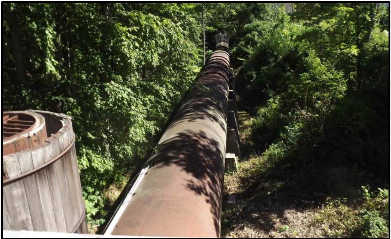
PHOTO 5-6 VIEW OF THE ABOVE GROUND STEEL PENSTOCK LOOKING UPSTREAM FROM POWERHOUSE
