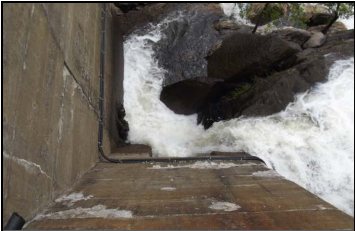
PHOTO 5-10 MINIMUM FLOW RELEASE THROUGH LOW LEVEL GATE AT NORTH DAM
