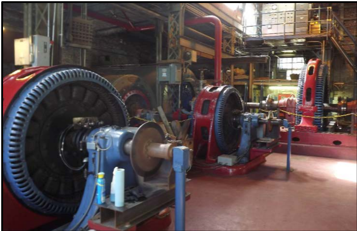
PHOTO 5-16 POWERHOUSE INTERIOR SHOWING HORIZONTAL TURBINE-GENERATOR UNITS
