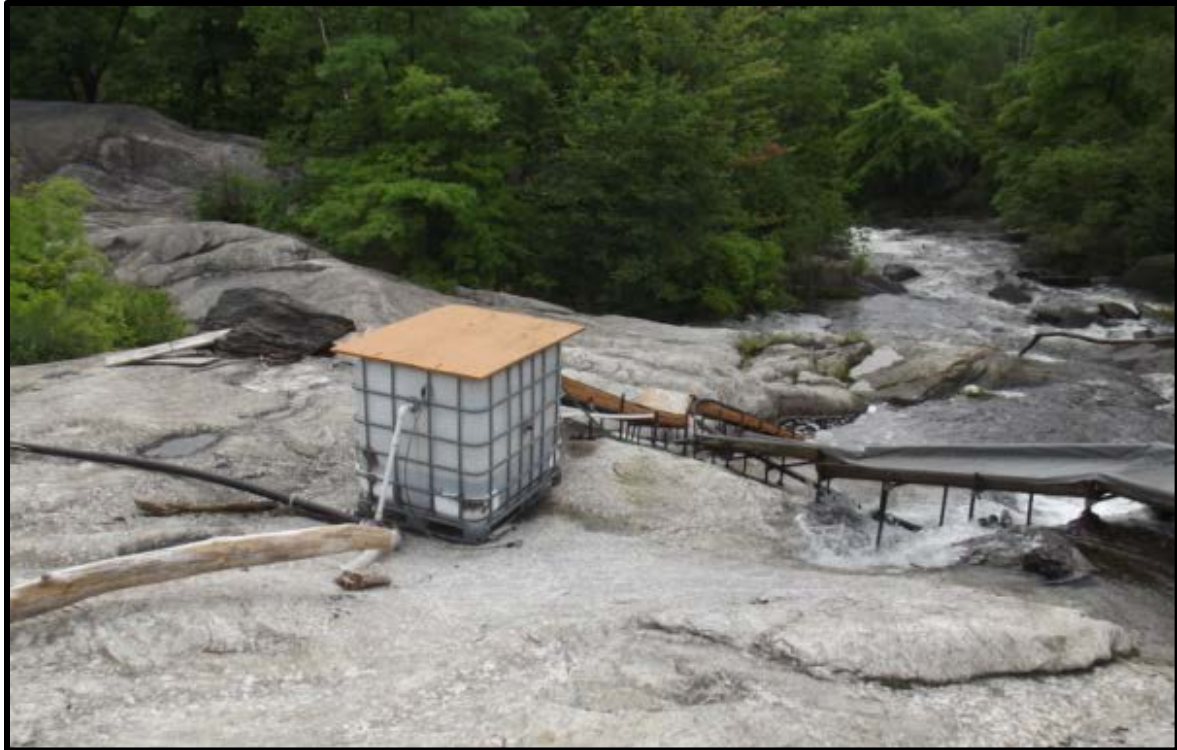
PHOTO 5-11 VIEW OF UPSTREAM EEL PASSAGE AND HOLDING TANK
