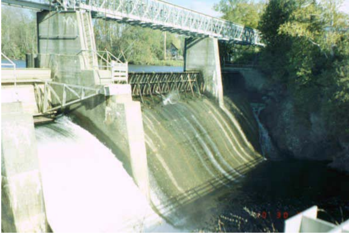
PHOTO 9 WEST SPILLWAY SECTION
