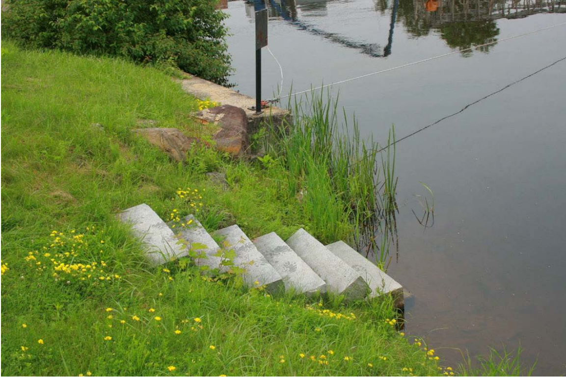
PHOTO 7 CANOE TAKE-OUT GRANITE STAIRS
