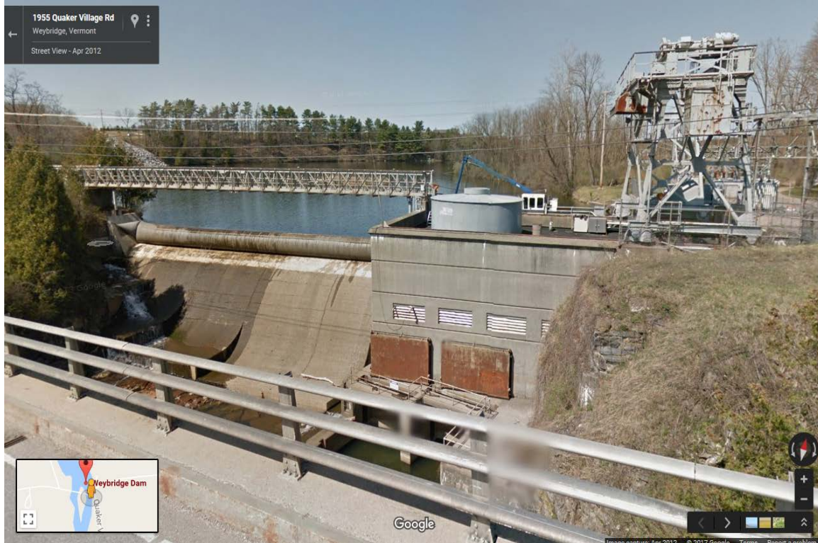
PHOTO 11 EAST SPILLWAY SECTION AND POWERHOUSE
