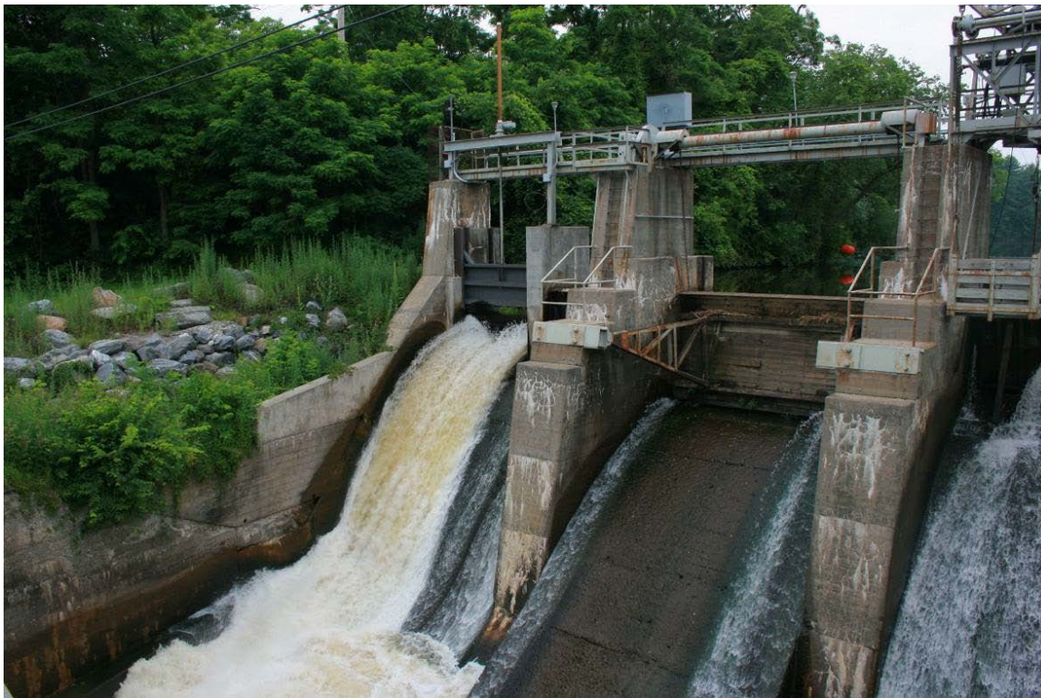
PHOTO 10 MINIMUM FLOW RELEASE FROM WEST SPILLWAY
