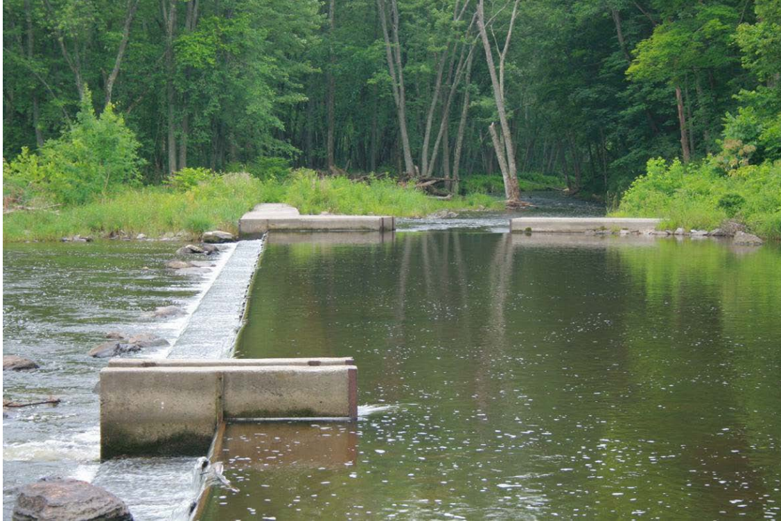
PHOTO 13 DIVERSION DAM AND FLOW CONTROL WEIR AT DOWNSTREAM END OF ROCK ISLAND
