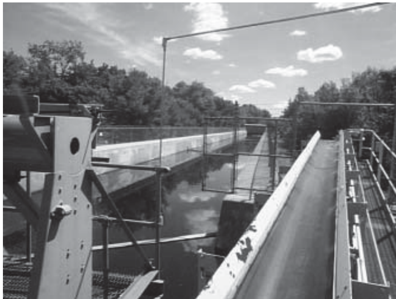
Figure 4 - Power Canal (looking upstream from bypass reach)
