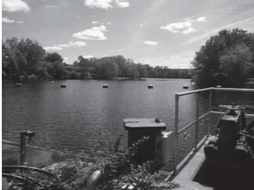
Figure 3 - Webster Reservoir (looking upstream from Webster dam)
