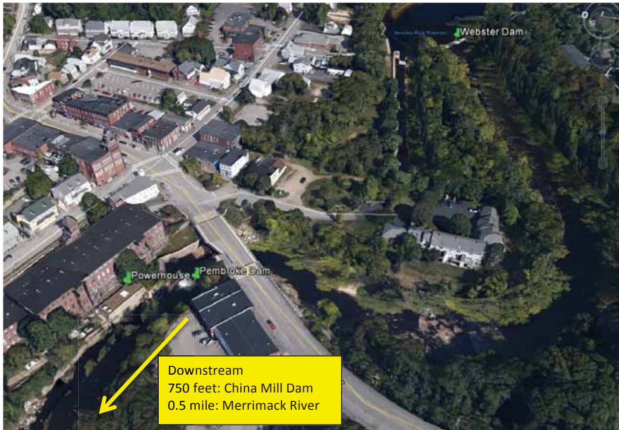
Figure 2 - Project Works at Webster-Pembroke
