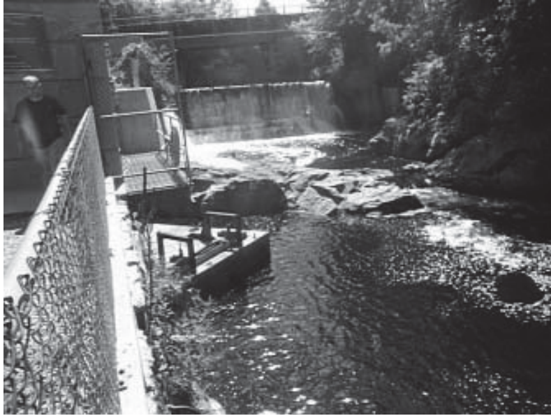
Figure 5 - Pembroke Dam releasing minimum flow (powerhouse on left)
