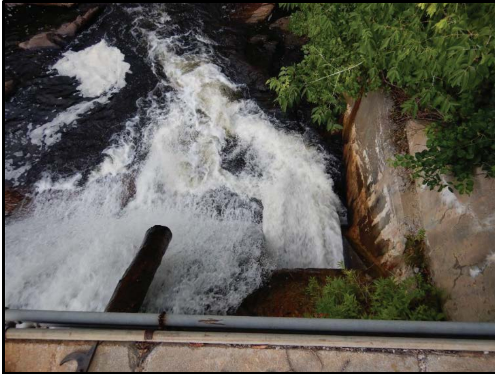
PHOTO 5-3 VIEW OF RIGHT SPILLWAY ABUTMENT AND SLUICE GATE OUTLET
