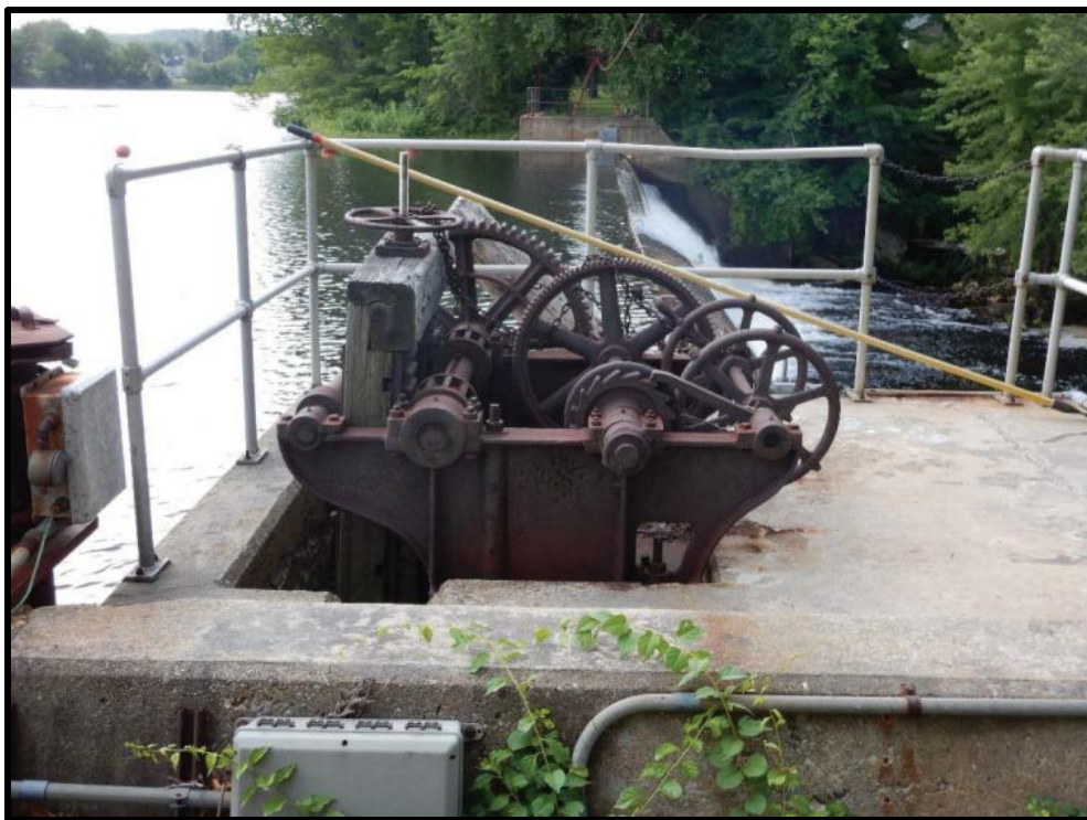
PHOTO 5-2 SLUICE GATE OPERATOR ON RIGHT ABUTMENT
