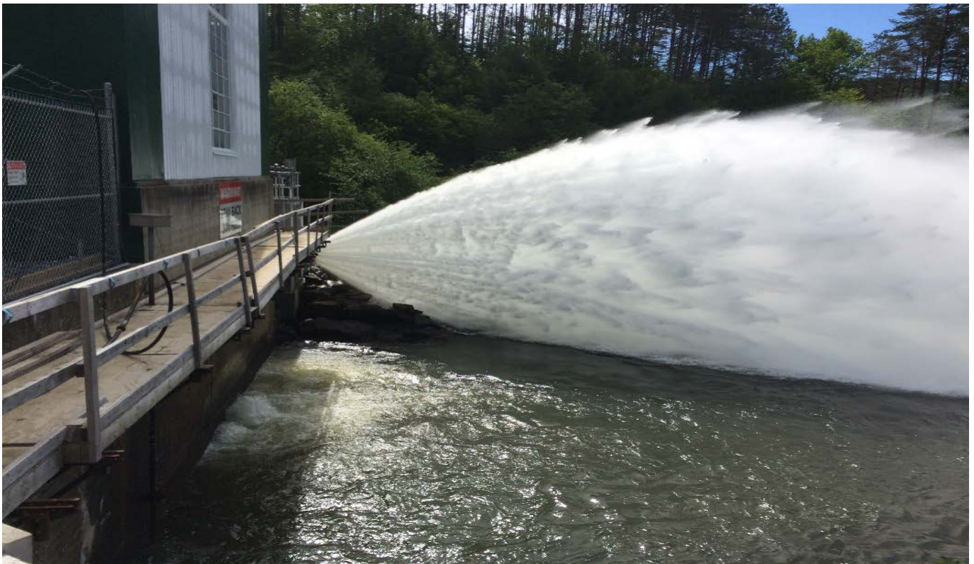
Figure 4 - Bypass Valve Discharge
