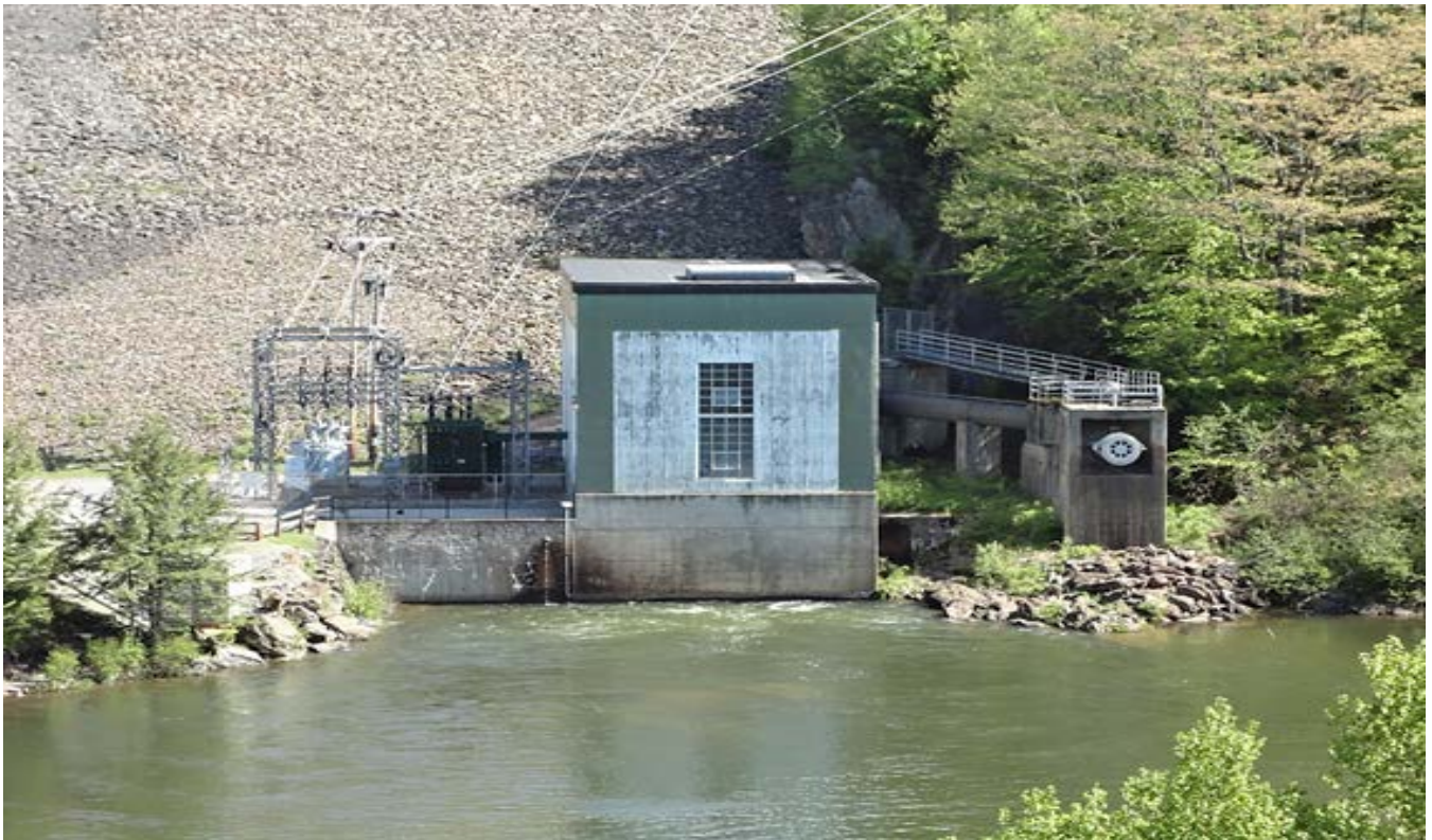
Figure 3 - Powerhouse, Bypass Valve and Substation Looking Upstream
