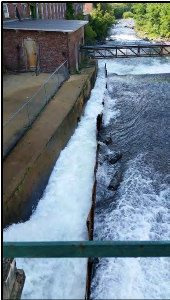
PHOTO 5-6 DOWNSTREAM FISH PASSAGE FACILITIES
