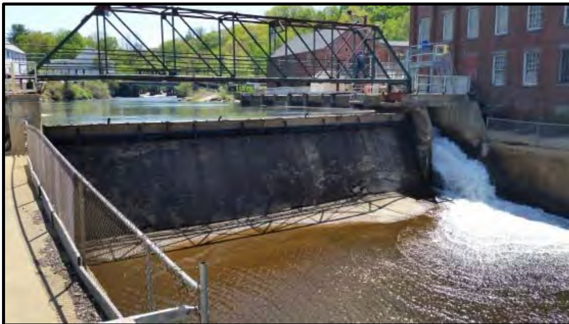
PHOTO 5-4 STEVENS MILL CONCRETE SPILLWAY WITH SLUICE GATE
