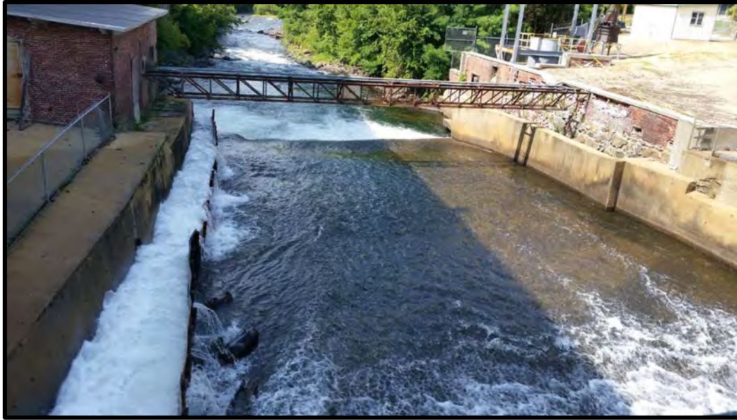
PHOTO 5-5 DOWNSTREAM FISH PASSAGE FACILITIES
