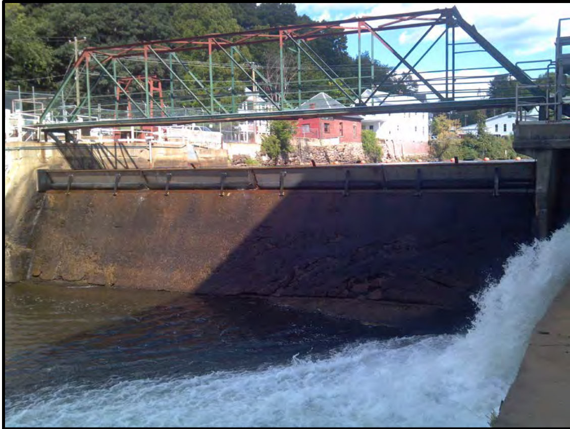
PHOTO 5-3 STEVENS MILL CONCRETE SPILLWAY
