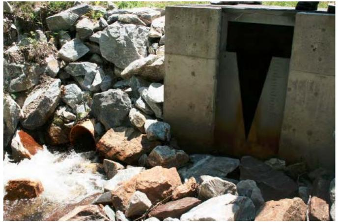
Figure 3 – Sucker Brook Diversion Dam Release Structure
