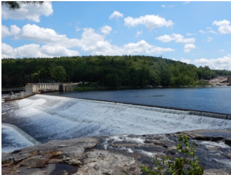
Rumford Falls Middle Dam and Impoundment (Zone 3)
