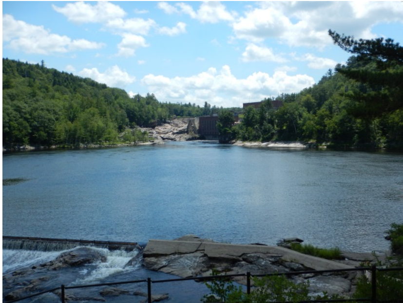
Rumford Falls Middle Dam Impoundment (Zone 3)
