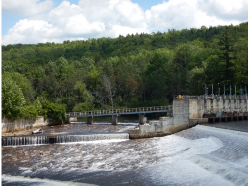
Rumford Falls Middle Dam Canal
