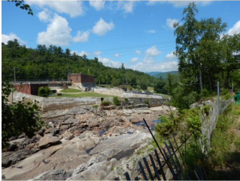
Rumford Falls Upper Dam and Powerhouse Bypass Reach (Zone 2)
