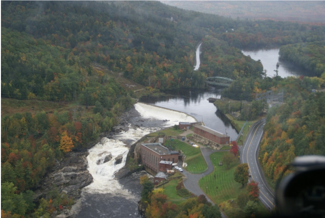
Upper Dam and Powerhouse, Impoundment and Bypass Reach (Zone 1 and 2)
