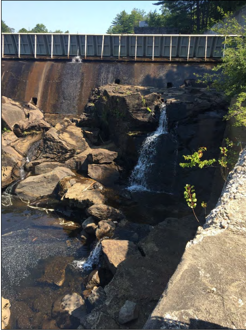
Figure 3. Area downstream of Eastman Falls spillway targeted for installation of an interim upstream eel trap. Collection tank will be installed at upper elevation with collection pipe descending around into watered habitat in vicinity of natural leakage. Natural leakage will be supplemented with additional attraction flow from headpond.
