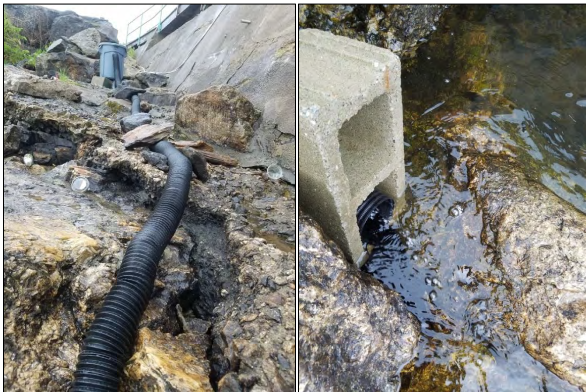
Figure 4. Proposed Eastman Falls interim eel trap design based on traps installed at Garvins Falls. Left panel shows the collection tank and descending collection pipe. Right panel shows entrance to collection pipe with flared netting material extending out into watered habitat.
