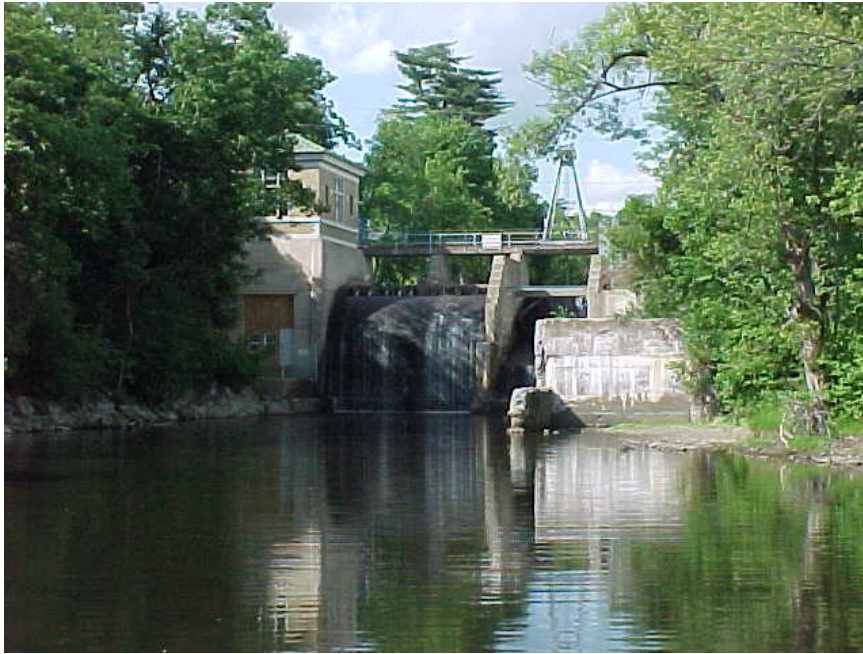
Figure 3. View of the dam from across the tailpool.
