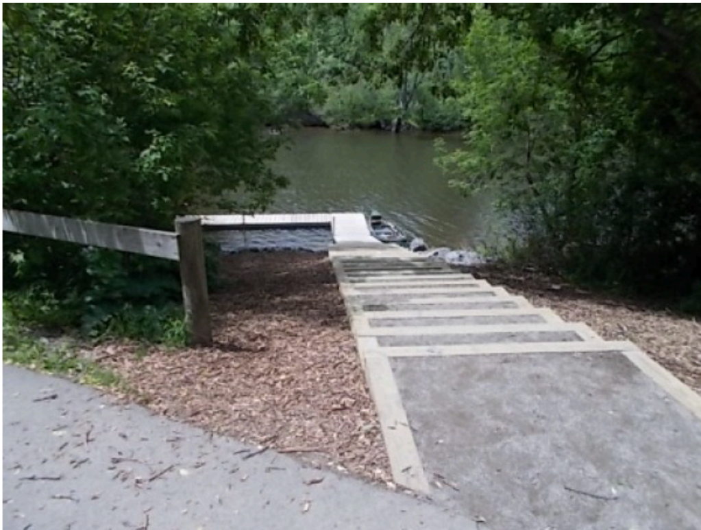
Figure 8. North Street Carry-in Boat Launch and Dock.
