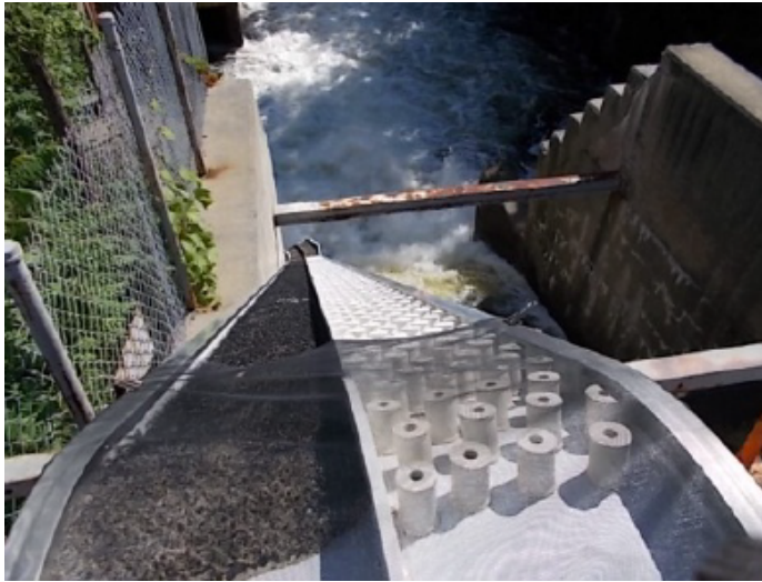
Figure 6. View down the eel ladder from the deck.
