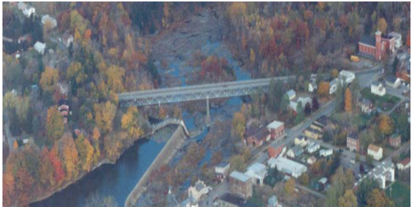
Figure 3 - Schaghticoke Spillway and Canal
