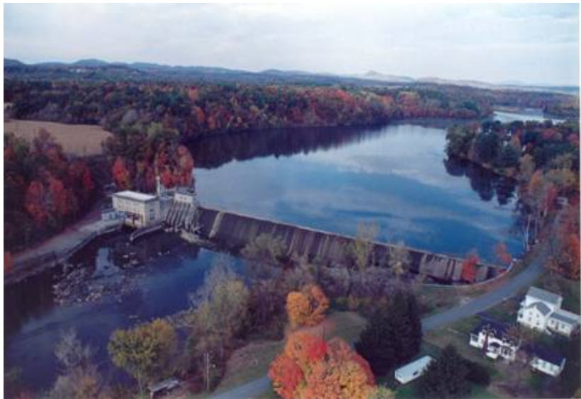
Figure 2 - Johnsonville Dam and Powerhouse
