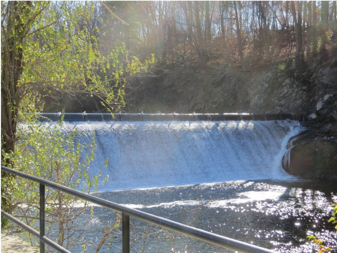
**Figure 7. The crest gates on top of the dam control spill across the length of the dam, maximizing air entrainment increasing dissolved oxygen content of downstream river flow.**
