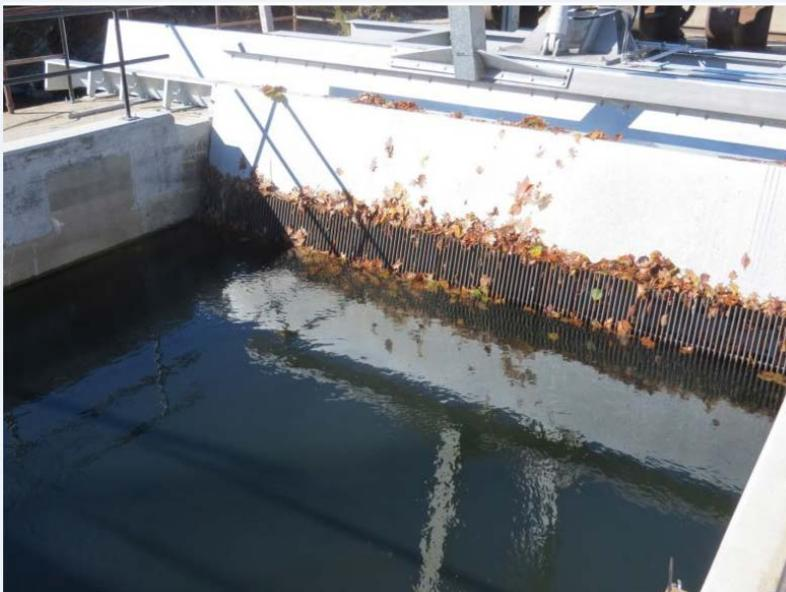
**Figure 9. The close spacing of vertical bars on the trashrack prevent large fish from entering the turbine.**
