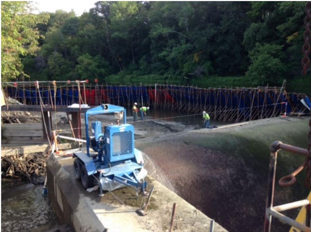
**Figure 8- Remediation of the impoundment Zone and removal of contaminated substrate.**
