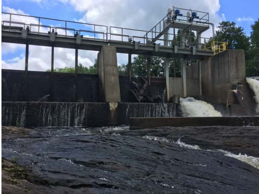
Figure 3 - Downstream face of spillway with 20 cfs fish movement facility
