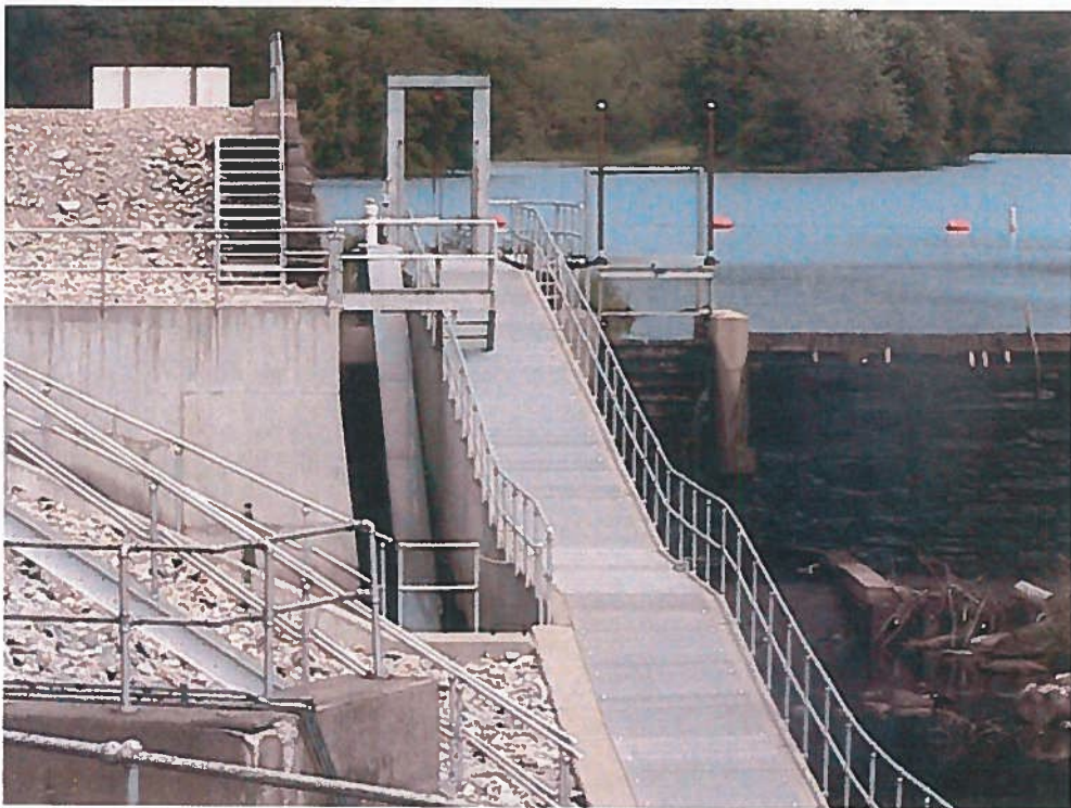
Photo 6: Occum Eel Ladder and Denil Fish Ladder
