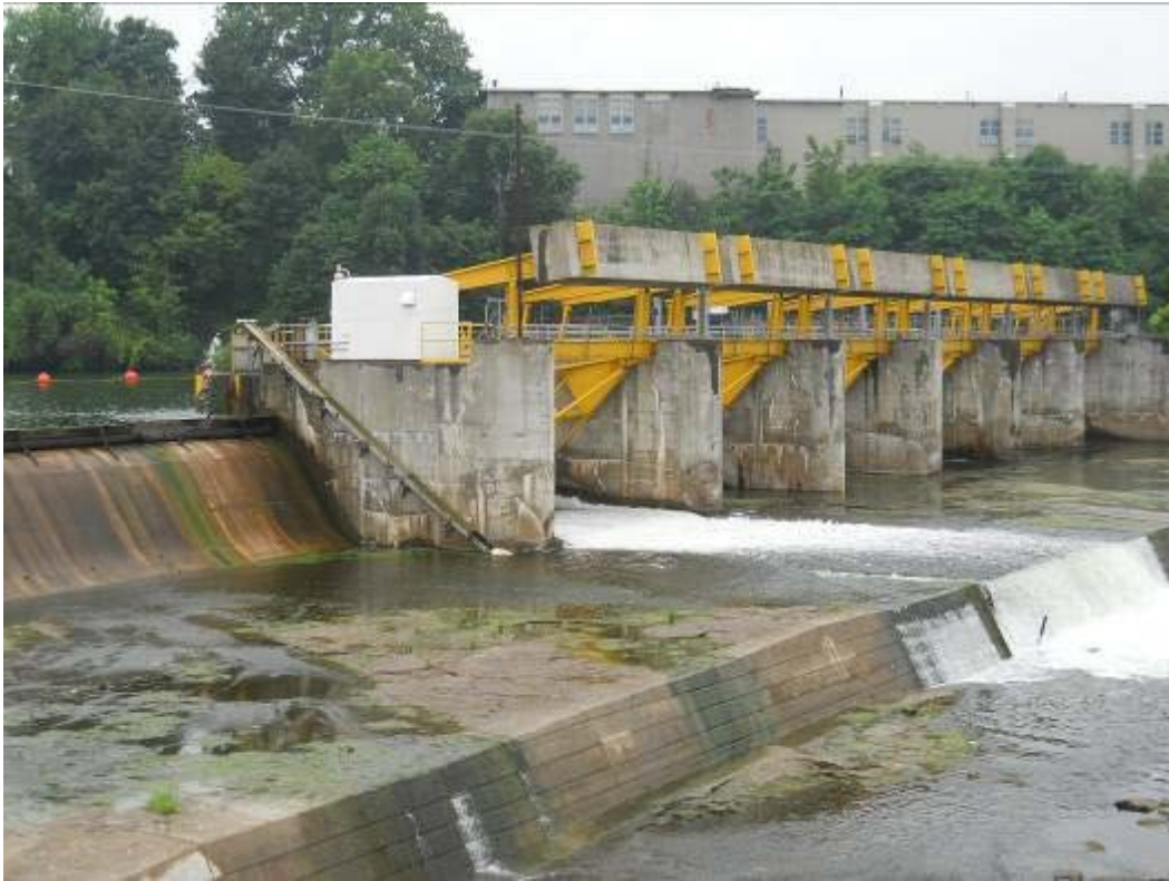
Figure 2 - Upstream eel conveyance system (adjacent to Tainter gate)
