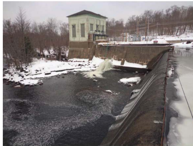
Figure 3 - Lower Newton Falls Minimum Flow Outlet
