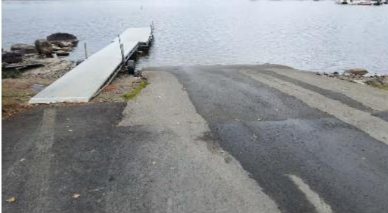
Figure 6: South Twin Lake boat ramp
