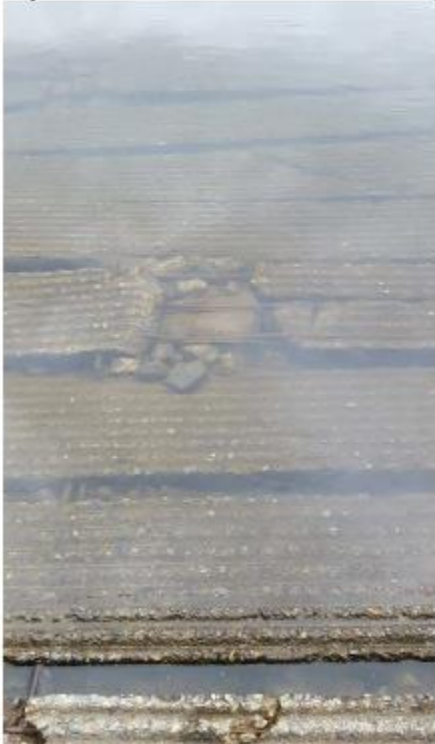
Figure 9: Millmocket Lake Boat Ramp exposed rebar
