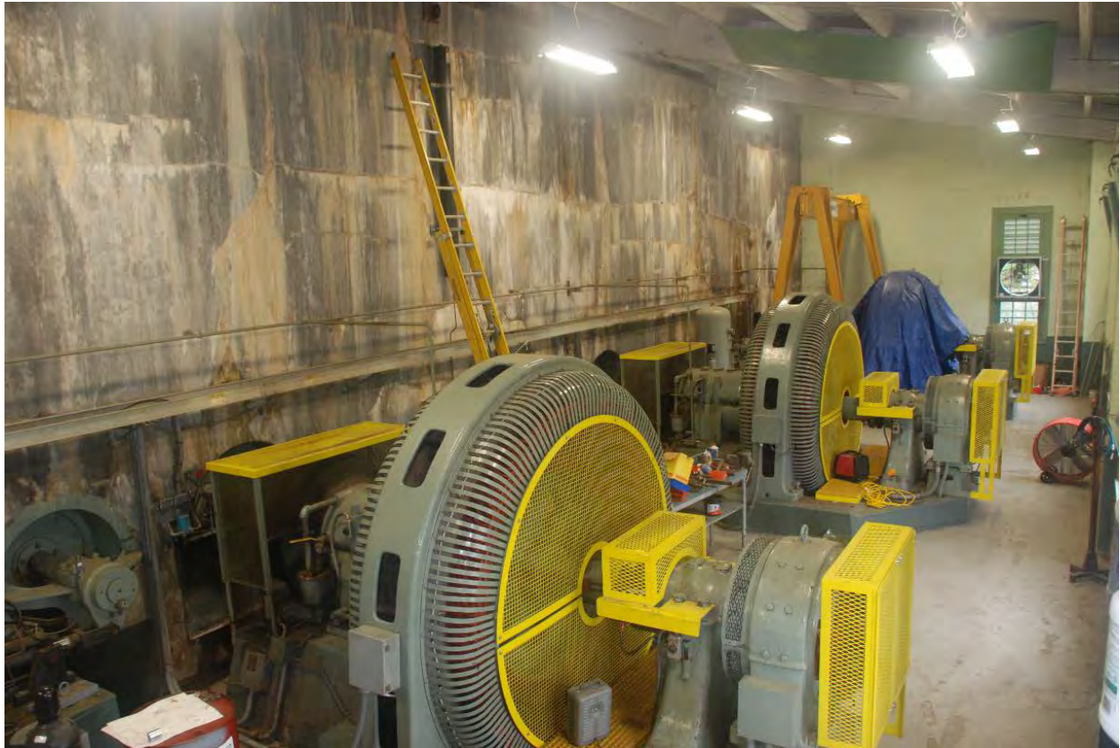
Figure 5 - View of Three Francis Turbines/Generators
