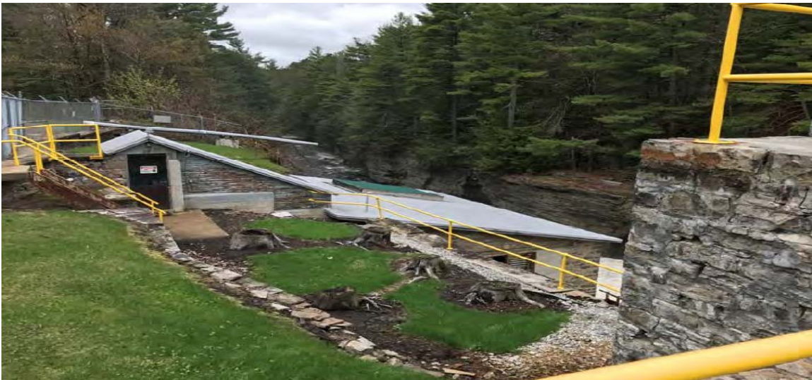
Figure 3 - Looking at Powerhouse from Intake
