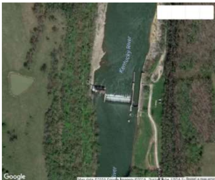
The Google Earth image above shows the powerhouse on the left, the dam in the center and the
