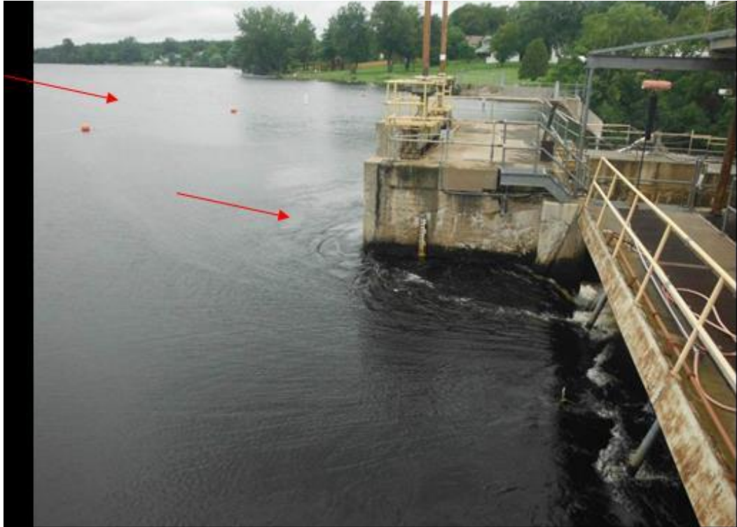
FIGURE 6: Norwood Development - Headpond staff gage (arrow) and intake to the power canal (Note: upstream boat barrier also visible).
