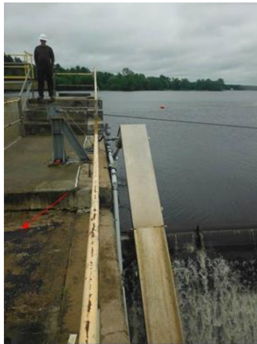
FIGURE 7: Norwood Development—Upstream eel passage ramp (Note: similar eel ramps in place at Norfolk, East Norfolk, and Raymondville Developments).
