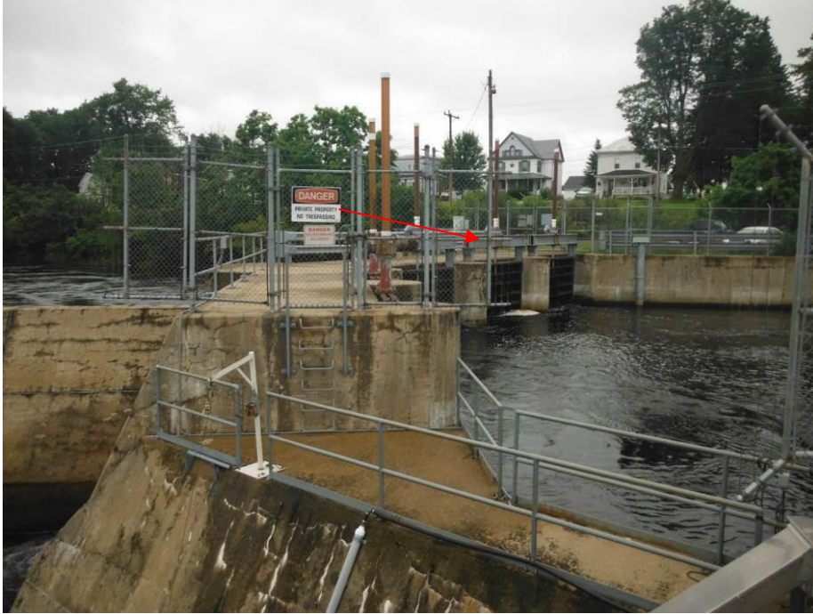
FIGURE 12: Norfolk Development—Headpond elevation sensor (arrow) (Note: similar sensors in place at Norwood, East Norfolk, and Raymondville Developments).
