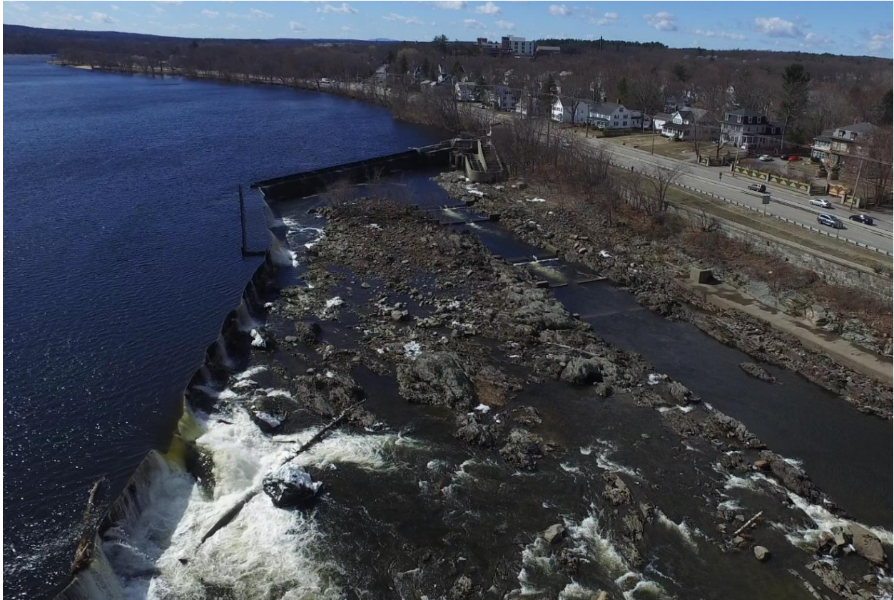
Figure 6 - Pawtucket Dam (Fish ladder in northwest abutment; weirs in river channel direct fish to ladder)
