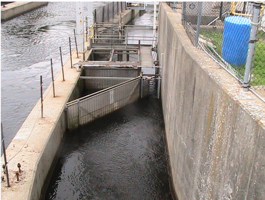
Photo 12H: Lawrence Upstream Fish Passage Exit Channel Trap
