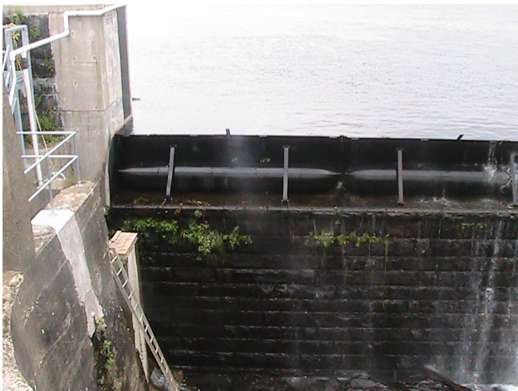
Photo 12C: Lawrence Dam Flashboards
