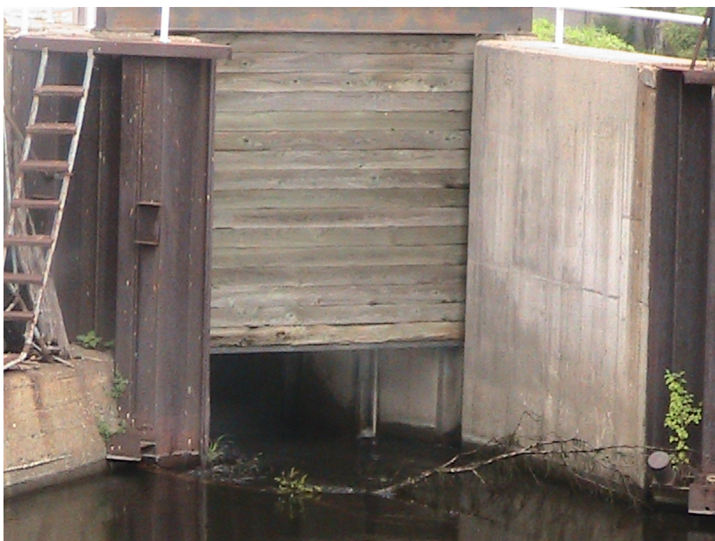
Photo 12D: Lawrence Downstream Fish Passage Entrance
