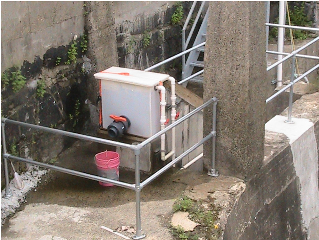
Photo 12J: Lawrence Upstream Eel Passage Collection Tank
