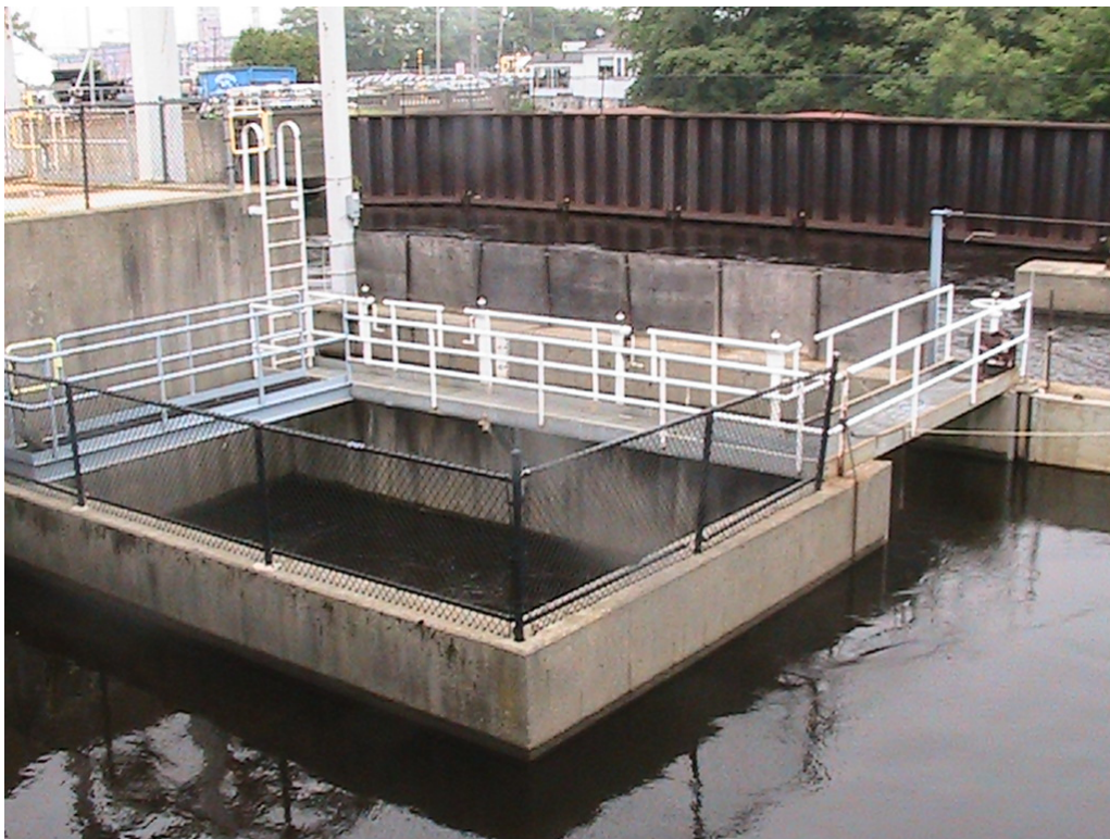
Photo 12M: Upstream Fish Passage Exit and Attraction Water inlet chamber
