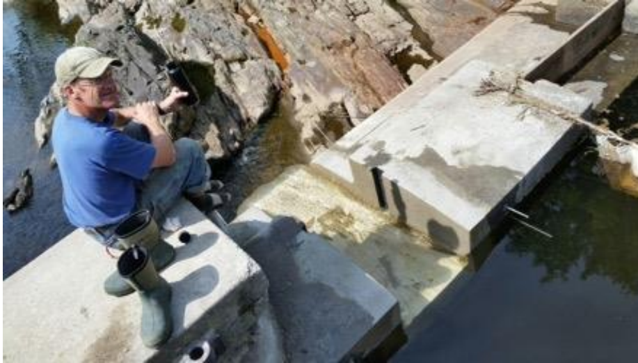
Figure 8 - Reconfigured Weir for Minimum Flow Passage
