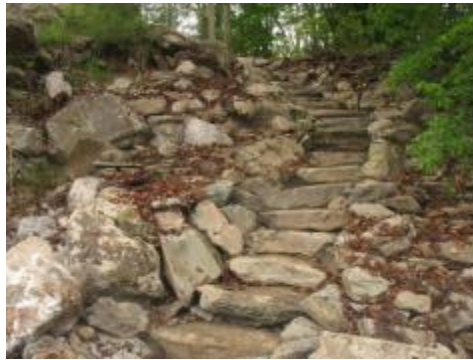
Figure 10 - Stone stairway to downstream access
