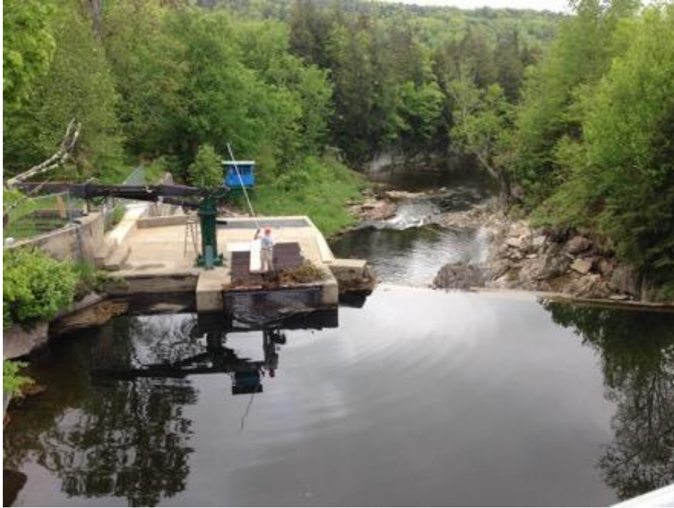
Figure 4 - Forebay and Powerhouse (looking downstream)
