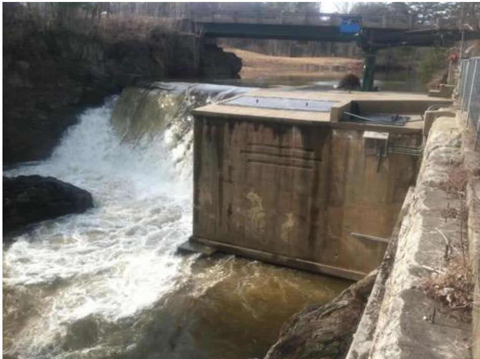
Figure 5 - Tailrace and Powerhouse (looking upstream)
