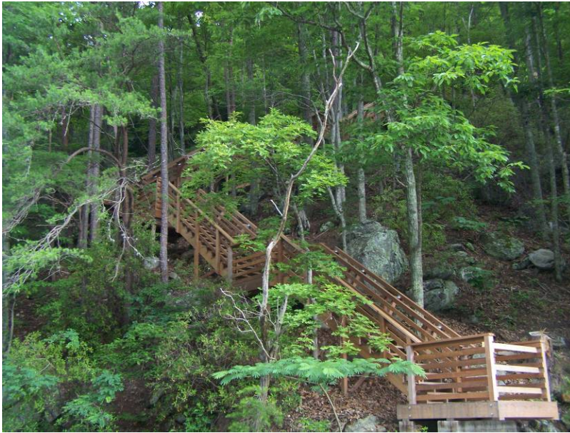
Calderwood Dam Portage Trail (upstream of dam)
