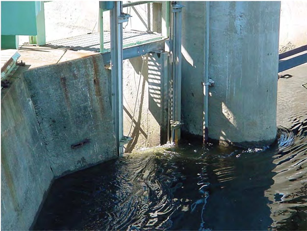
PHOTO 6 HOOKSETT FISH PASSAGE GATE
