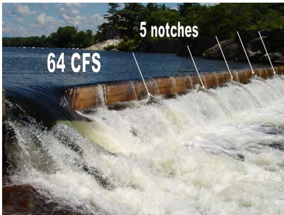
PHOTO 7 HOOKSETT SPILLWAY WITH 64 CFS
