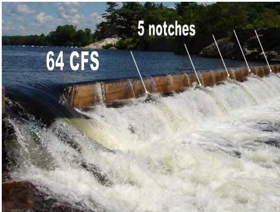
PHOTO 1 HOOKSETT SPILLWAY WITH 64 CFS
