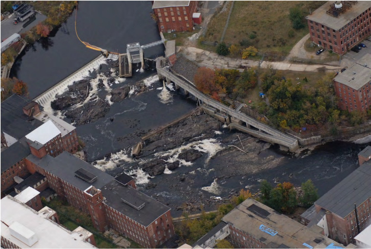
FIGURE 7. AERIAL OF PROJECT – WEST CHANNEL DAM
