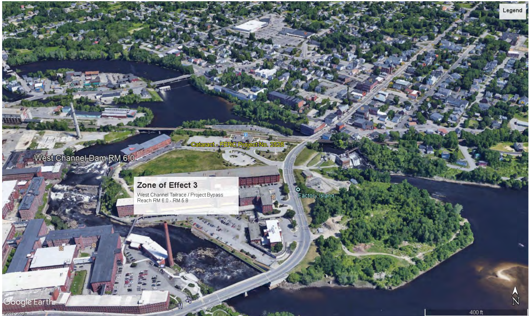
FIGURE 15. ZONE 3 – WEST CHANNEL TAILRACE/PROJECT BYPASS REACH
