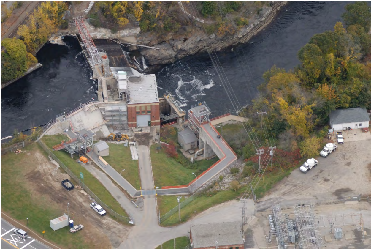
FIGURE 8. AERIAL OF PROJECT – EAST CHANNEL DAM
