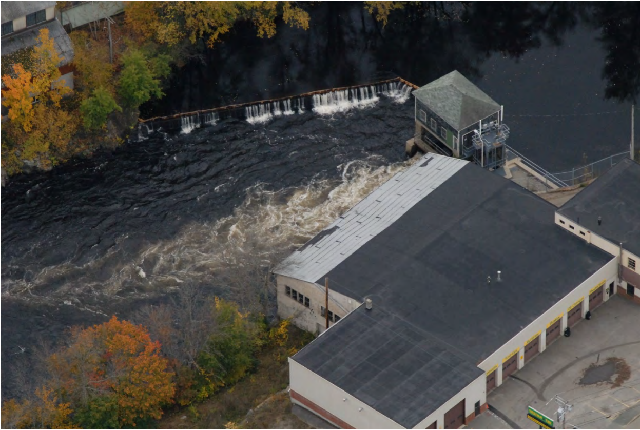
FIGURE 6. AERIAL OF PROJECT – BRADBURY DAM
