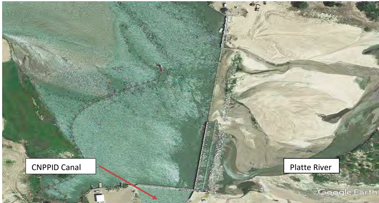
Figure 5 - Central Diversion Dam
