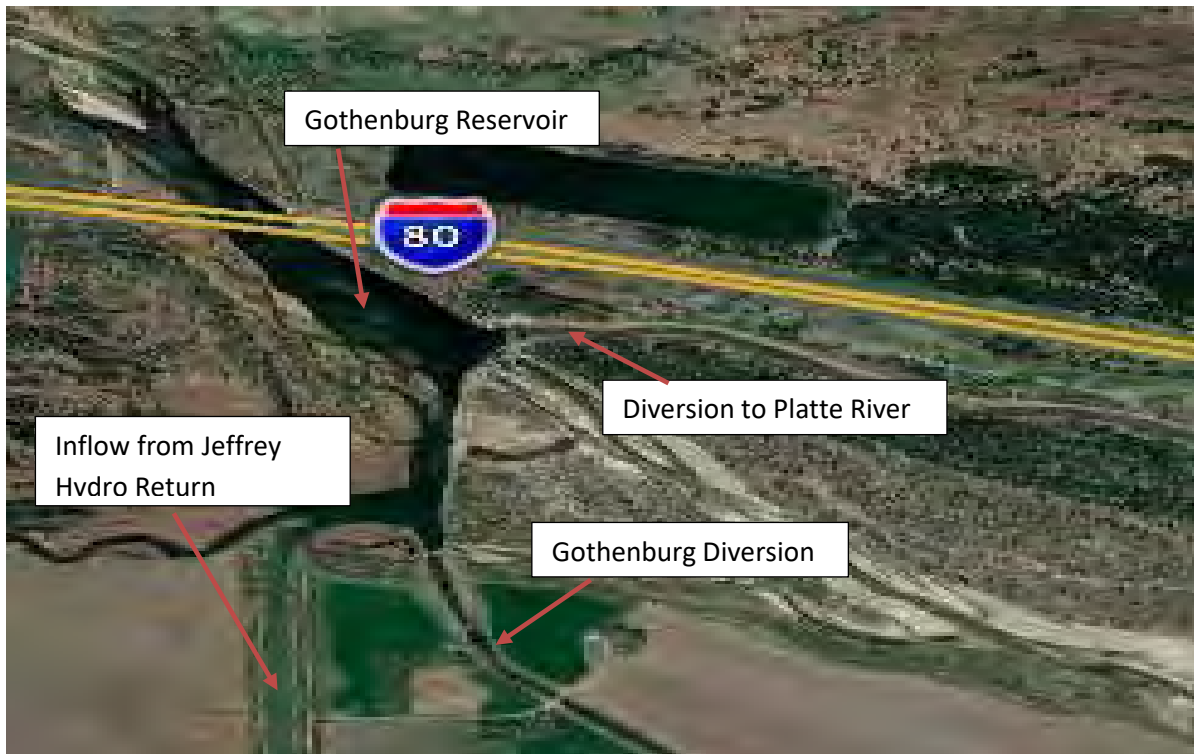
Figure 8 - Gothenburg Diversion Dam
