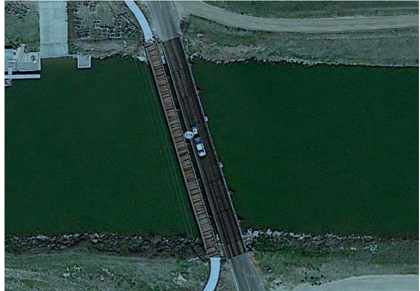
Figure 18 - Bridge across Outlet Canal
