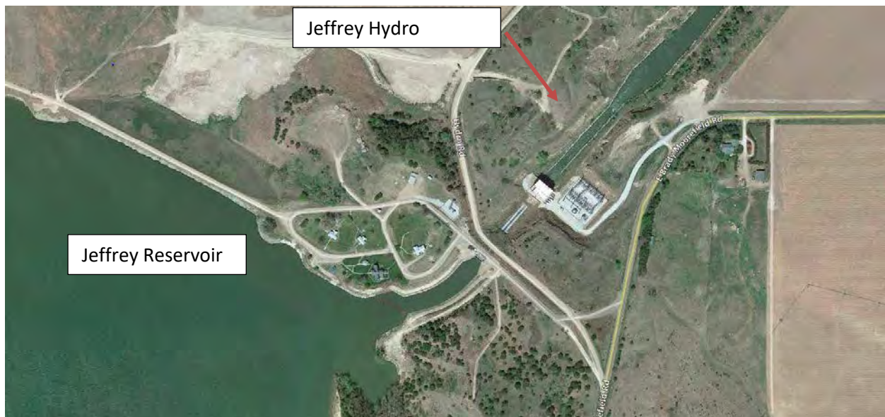
Figure 6 - Jeffrey Dam & Hydro
