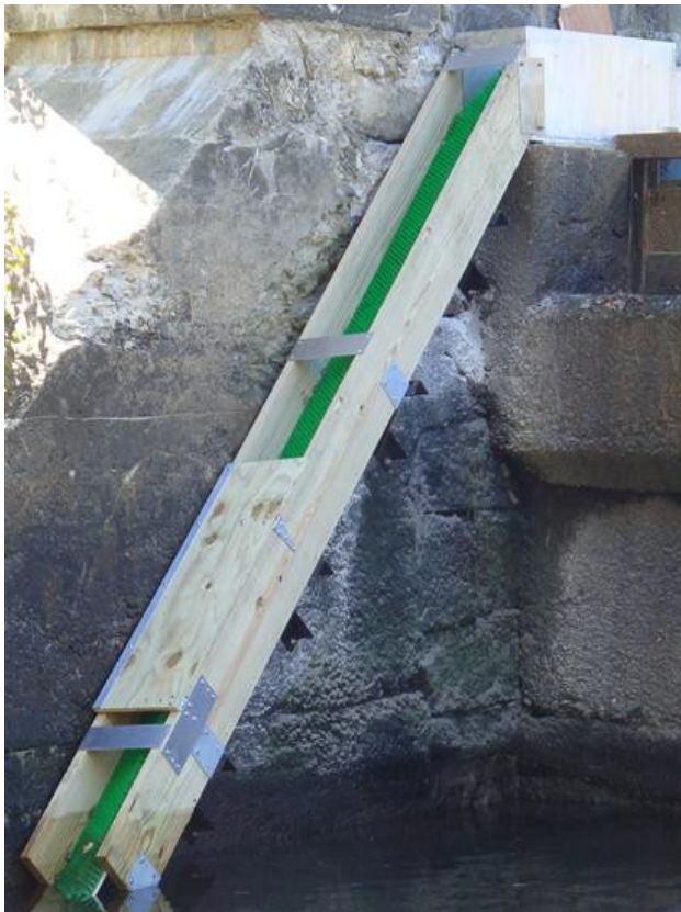
Figure 6. Ice House Upstream Eelway
