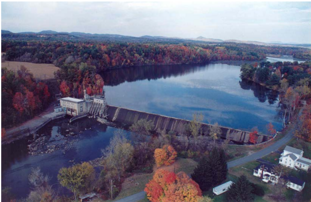
Figure 4 – Johnsonville Development Impoundment
