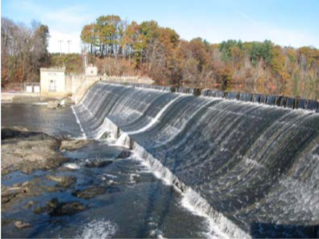
Figure 3 – Johnsonville Dam with Flashboards
