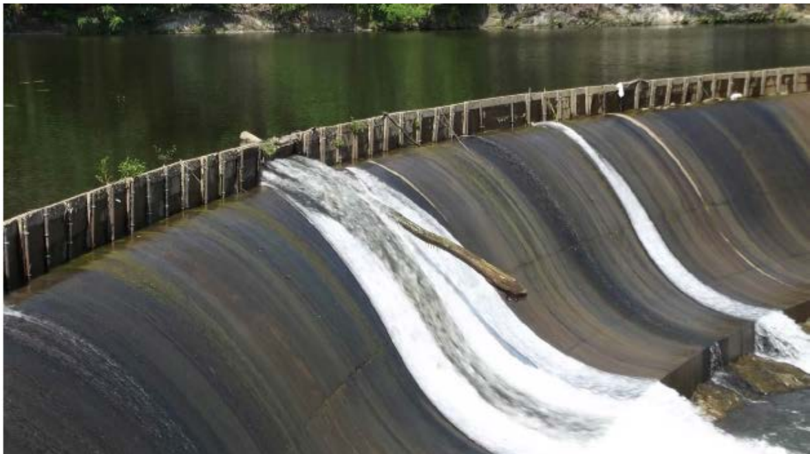
Figure 7 - Schaghticoke Development Dam Section with Wooden Flashboards
