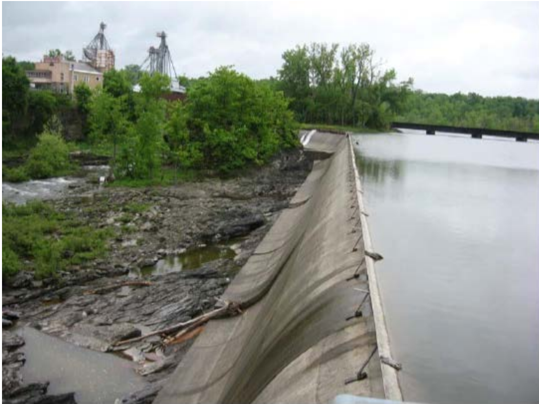
Figure 6 - Schaghticoke Development Dam Section with Pneumatic Flashboards
