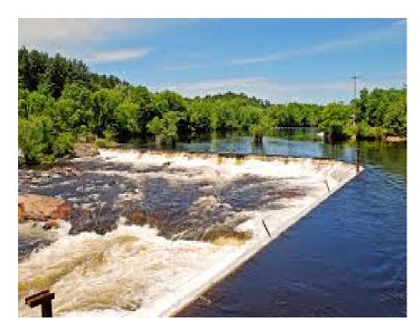
Photo 1: Masonry and Concrete Spillway
