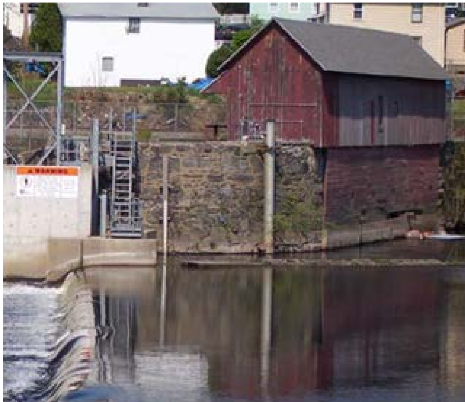
Photograph 2 – Power Canal Gatehouse
