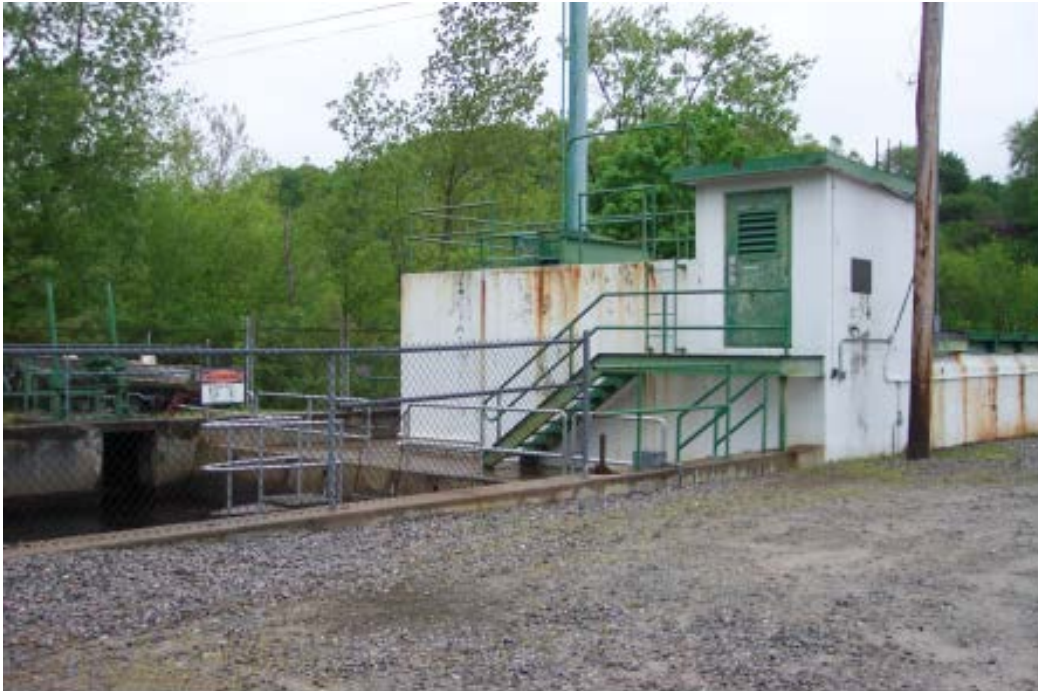
Photograph 3 - Tenth Street Station (intake side).
