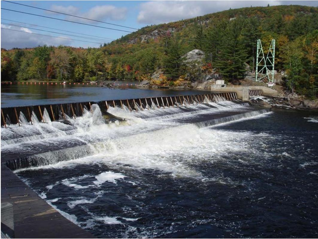
**PHOTO 4**      **VIEW OF LOWERED FLASHBOARD TO PROVIDE MINIMUM FLOW**
