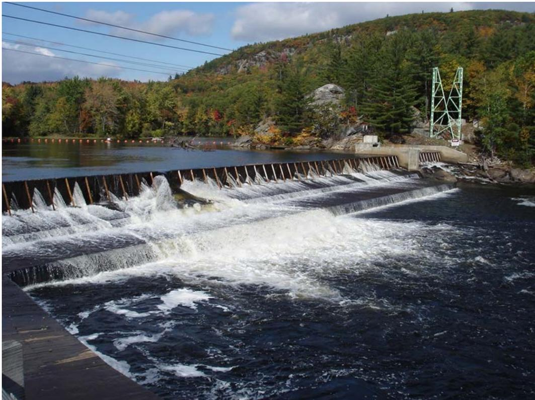
**PHOTO 8**      **VIEW OF LOWERED FLASHBOARD TO PROVIDE MINIMUM FLOW**
