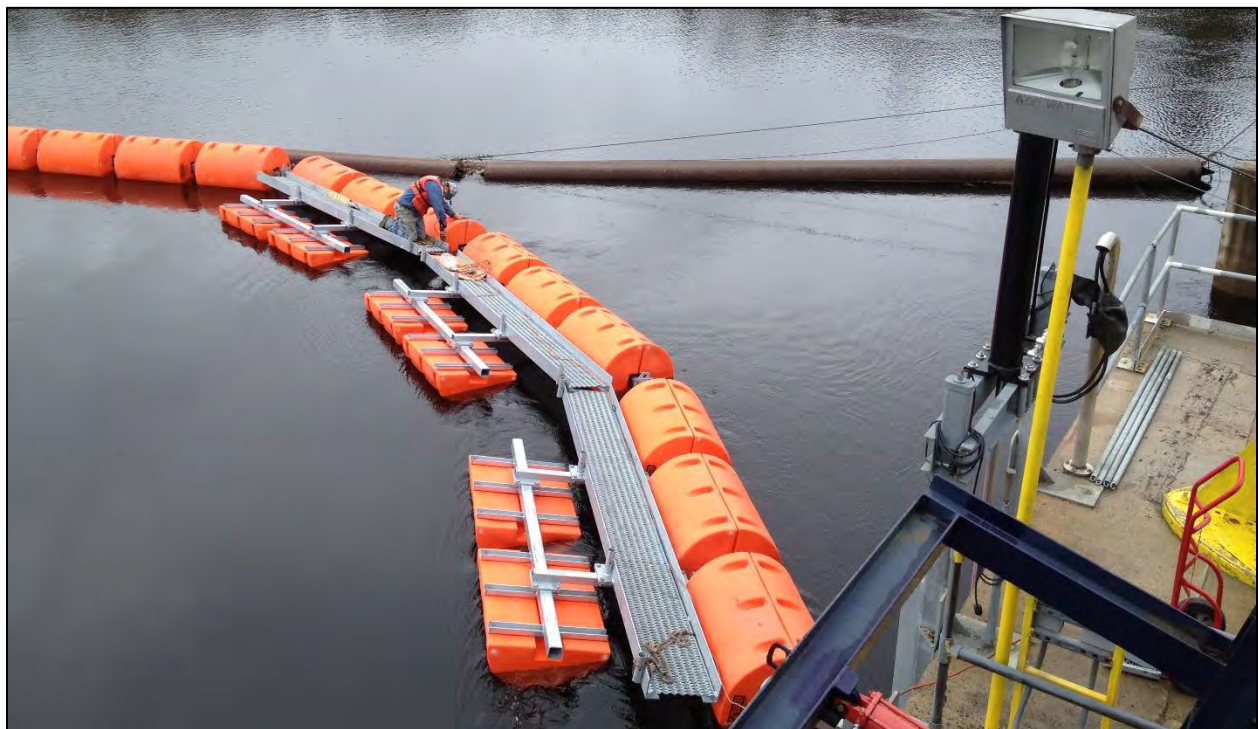
Figure 4. Angled boom installed upstream of fish passage
