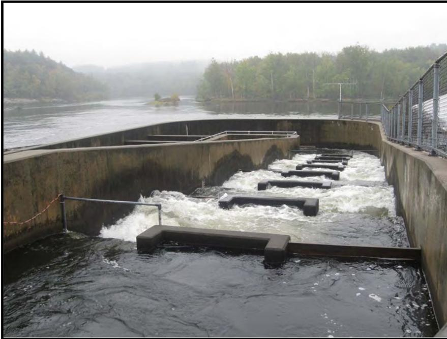
**Figure 6. Vernon fish ladder, lower section pool and weir configuration.**
