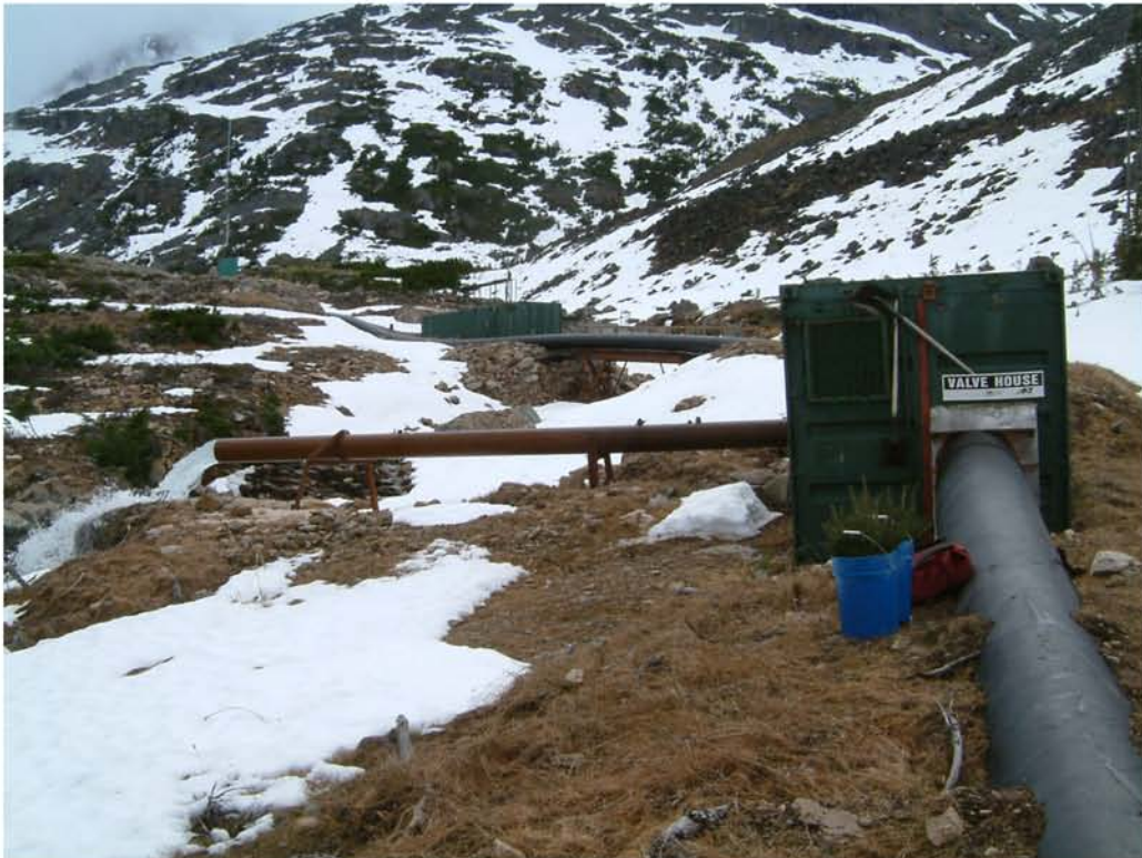
LOOKING UP TOWARD LAKE WITH VALVE HOUSE IN FOREGROUND BYPASSING FLOWS TO PITCHFORK FALLS STREAM; PUMPBACK HOUSE IN BACKGROUND AND GLACIER MORaine AT UPPER RIGHT
