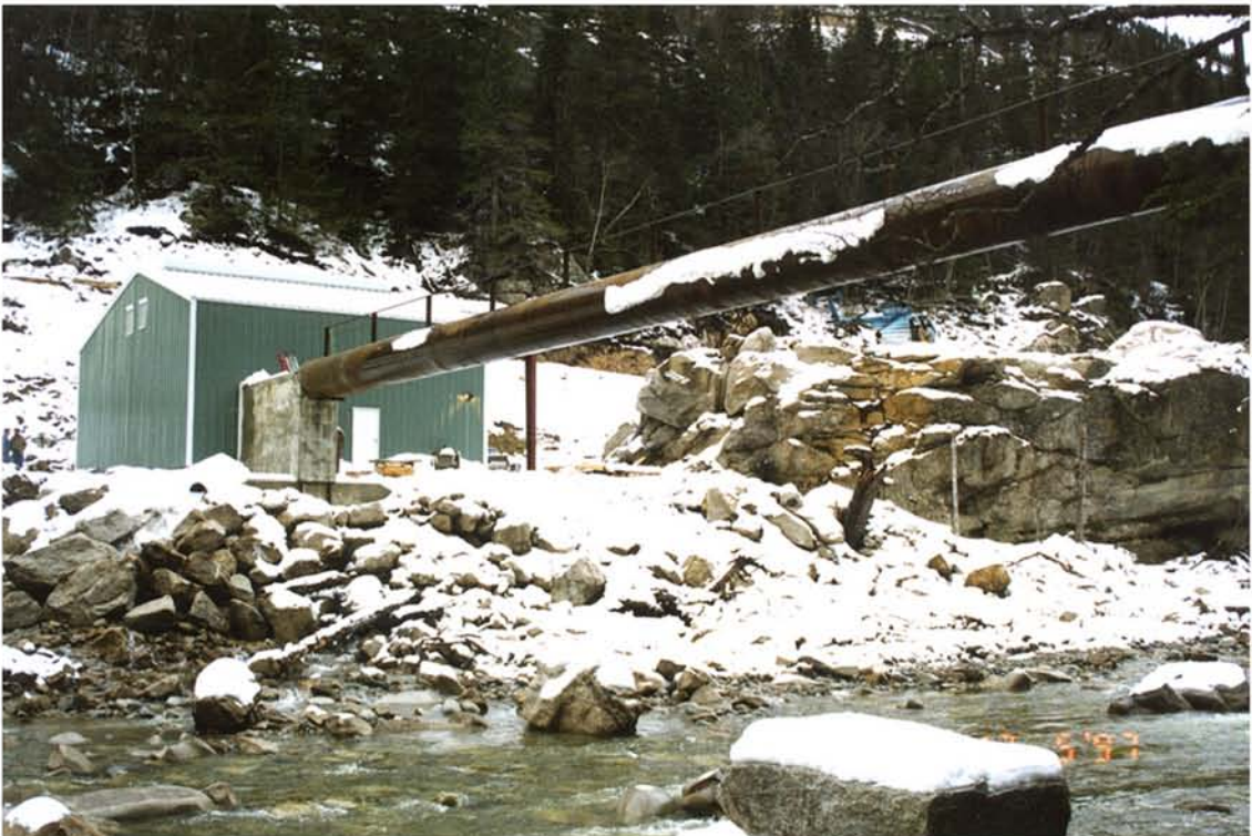
VIEW OF THE PENSTOCK CROSSING THE SKAGWAY RIVER TO THE POWERHOUSE
