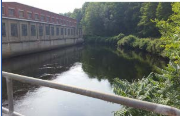
Powerhouse and Intake
