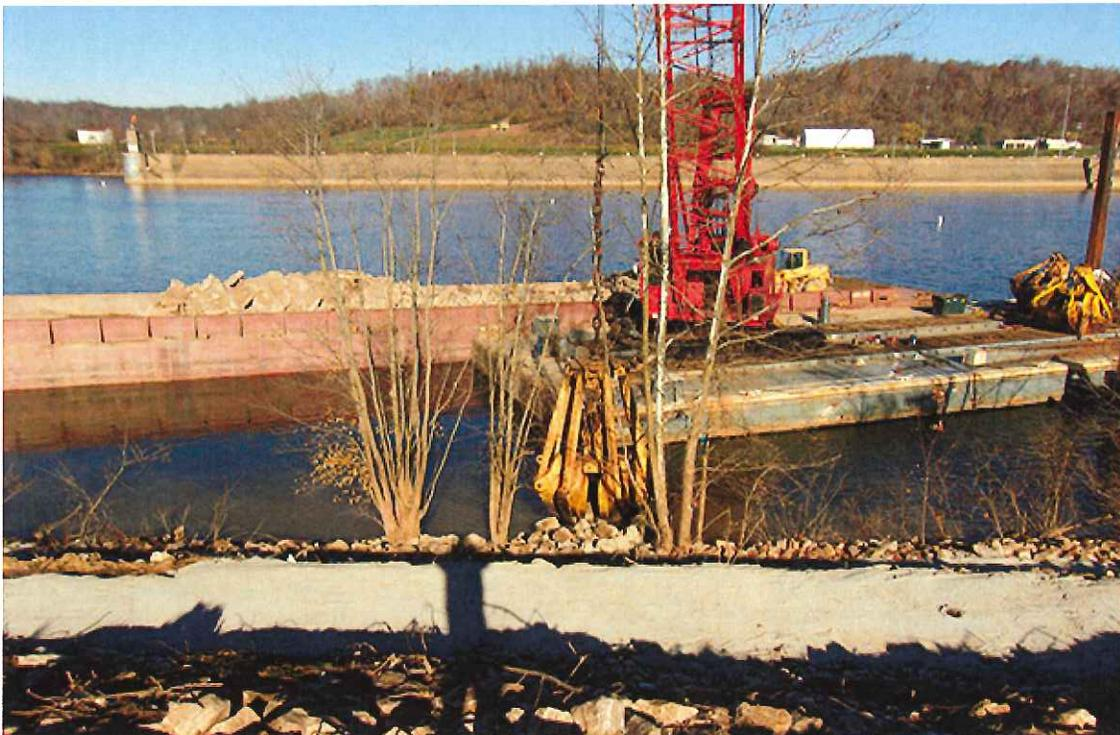
**Photo 12** November 2015 Placing Riprap on Downstream Slope (Photo Courtesy of MWH)
