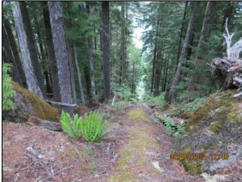
Buried penstock at crest of mountain just beyond standpipe (left) and along penstock corridor (below).
