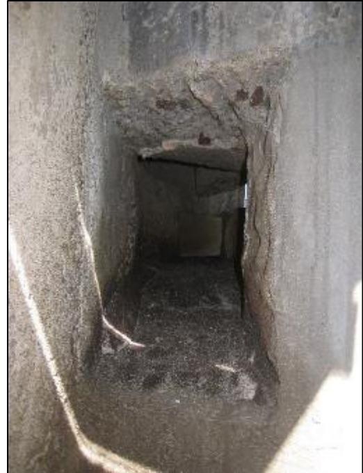
Water bypass channel of 1 CFS, above and right. Notice little to no water flowing over weir wall due to low flows in Falls Creek.
