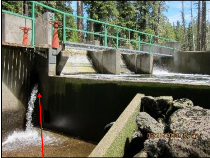
Water bypass channel of 1 CFS, above and right. Notice little to no water flowing over weir wall due to low flows in Falls Creek.
