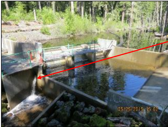
Minimum flows during operation
