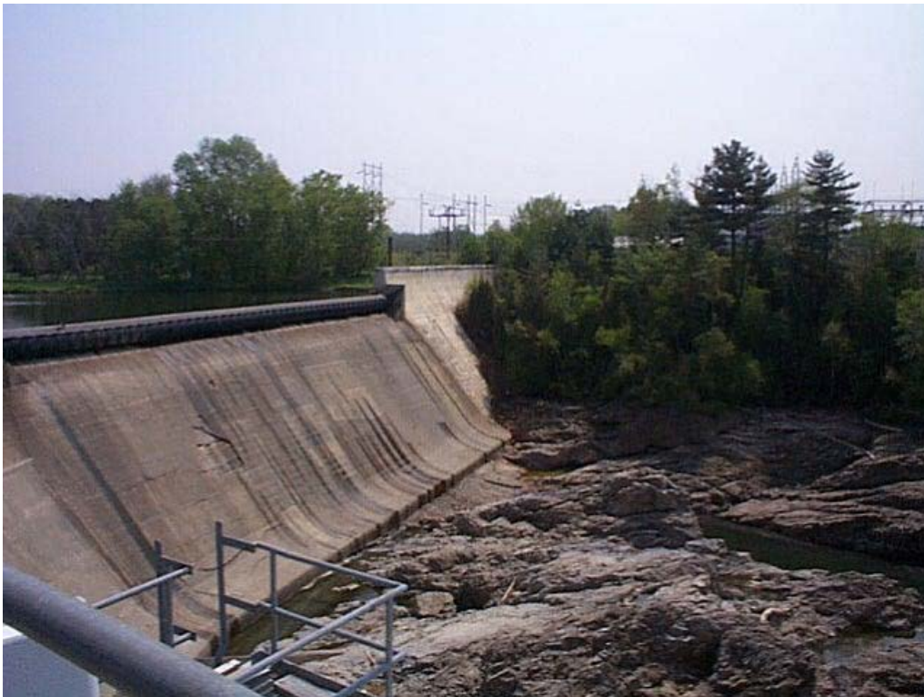
Side view of the dam
