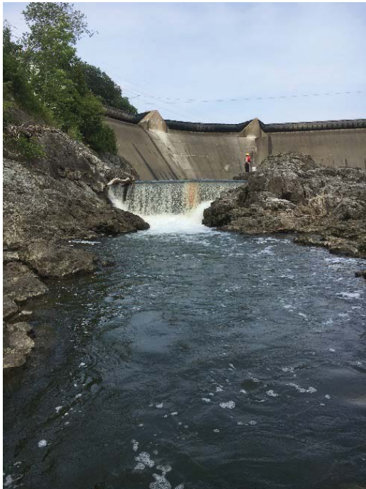
PHOTO 6 FLOW EXITING THE MODIFIED WEIR AT APPROXIMATELY 100 CFS FISHWAY DISCHARGE (COURTESY OF VTFW)
