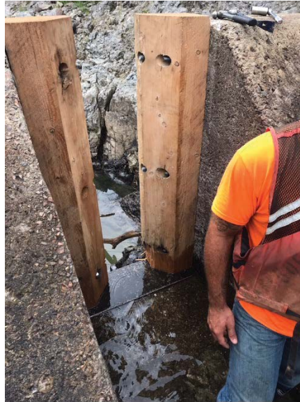
PHOTO 1 TEMPORARY BROAD-CRESTED WEIR (DEWATERED POST CONSTRUCTION)
