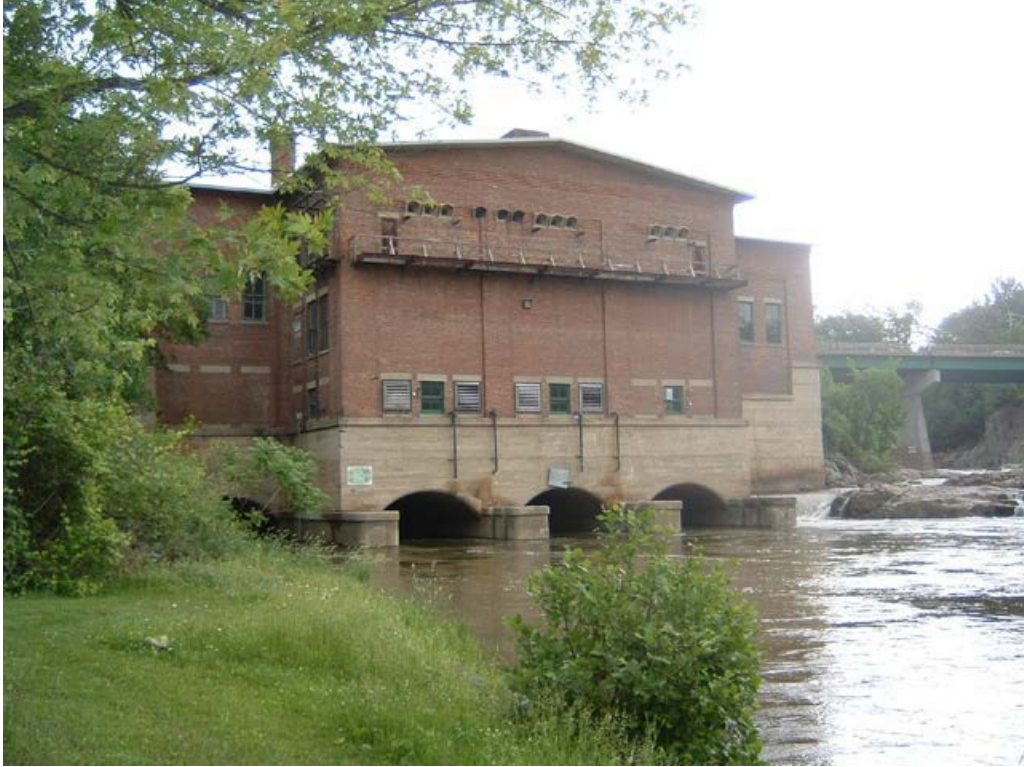
Upstream view of the powerhouse
