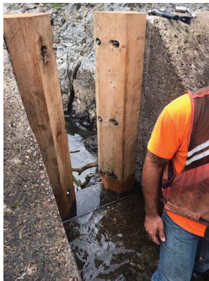
PHOTO 1 TEMPORARY BROAD-CRESTED WEIR (DEWATERED POST CONSTRUCTION)
