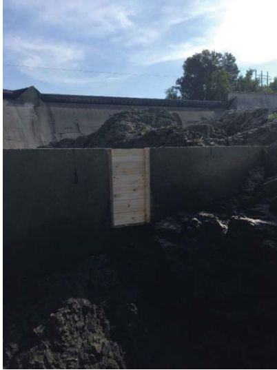
PHOTO 3 DOWNSTREAM WEIR PLUGGED TO TEMPORARILY RAISE PLUNGE POOL ELEVATION (DE-WATERED)
