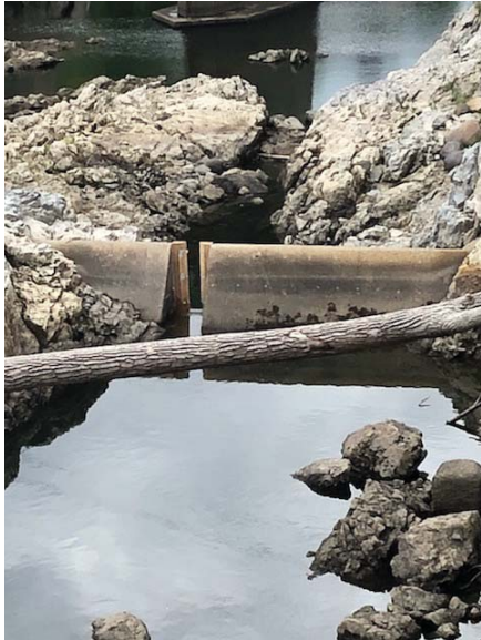
PHOTO 1 TEMPORARY BROAD-CRESTED WEIR (DEWATERED POST CONSTRUCTION)
