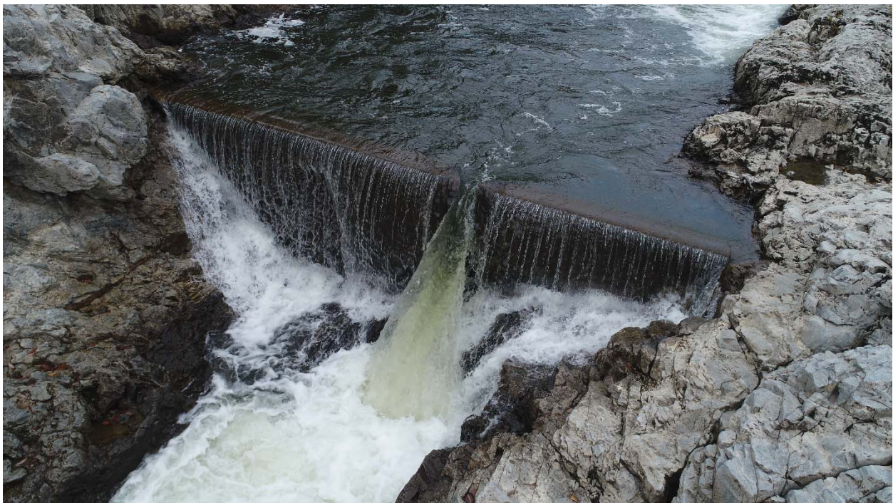
PHOTO 2 TEMPORARY BROAD CRESTED WEIR (IN OPERATION)
