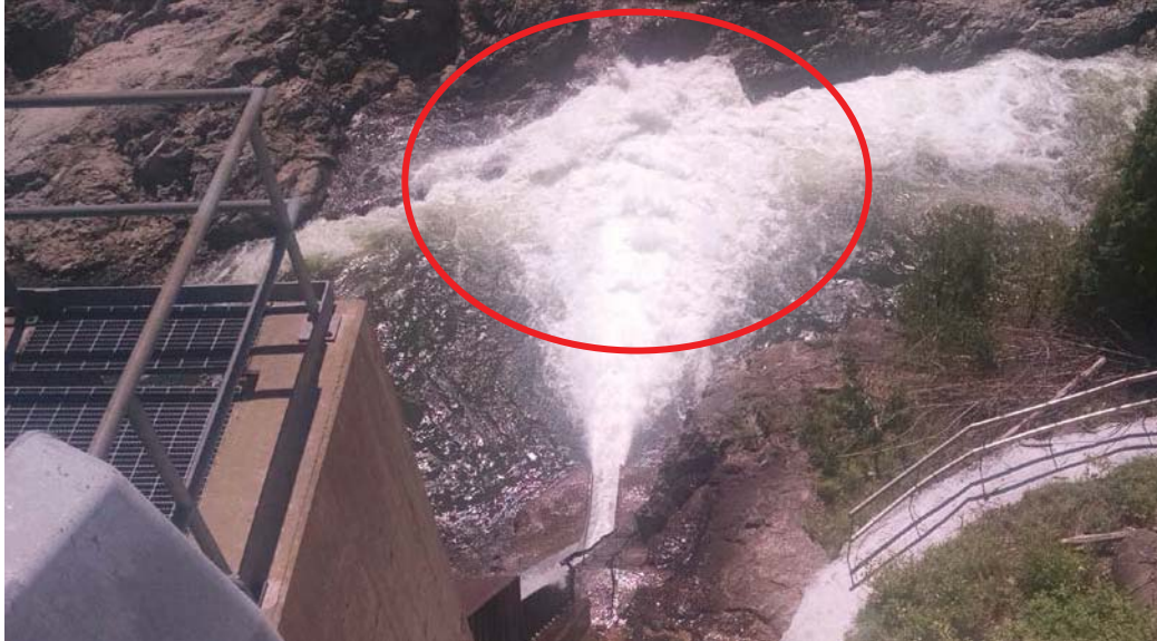
PHOTO 1 FLOW OF APPROXIMATELY 100 CFS DISCHARGED FROM DOWNSTREAM FISHWAY UNDER ORIGINAL PLUNGE POOL CONDITIONS
