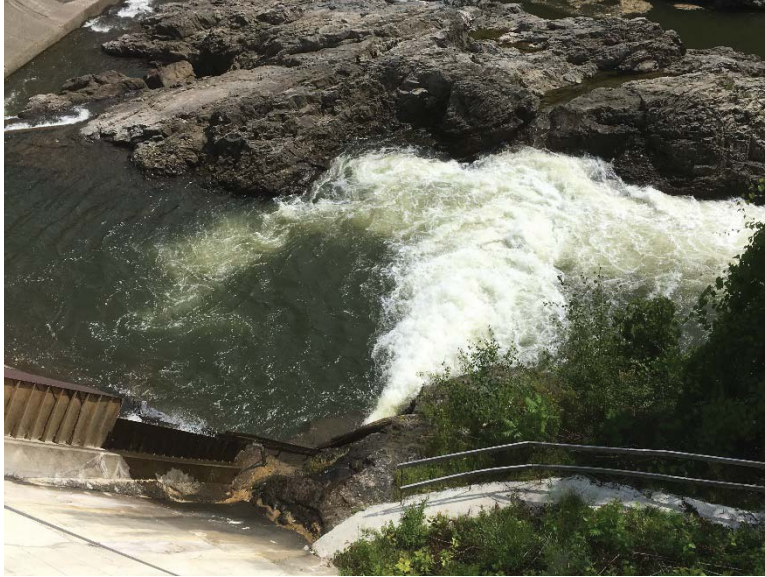
PHOTO 4 DOWNSTREAM FISHWAY DISCHARGE AT APPROXIMATELY 100 CFS WITH ELEVATED POOL (COURTESY OF VTFW)
