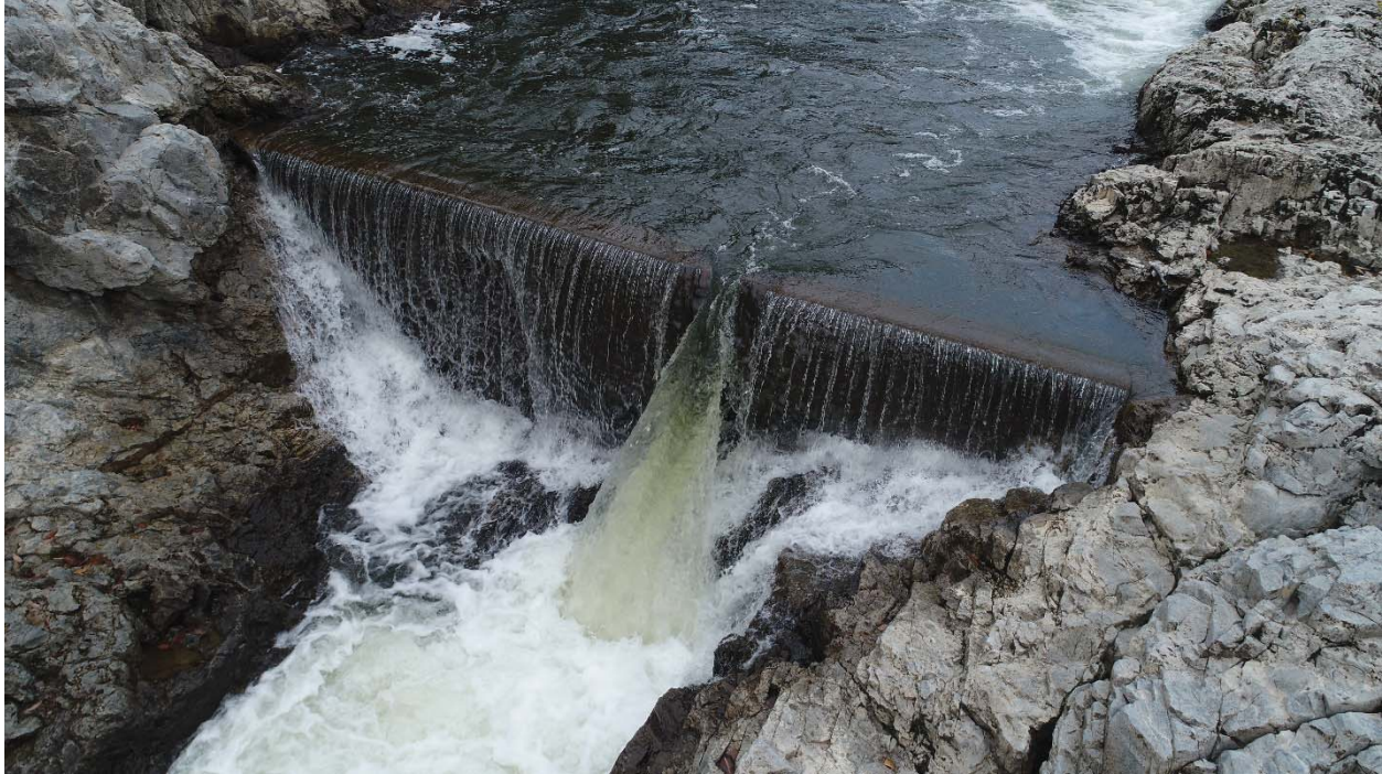
PHOTO 2 TEMPORARY BROAD CRESTED WEIR (IN OPERATION)
