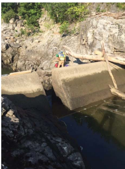
PHOTO 2 ORIGINAL DOWNSTREAM WEIR CONDITION (DE-WATERED)
