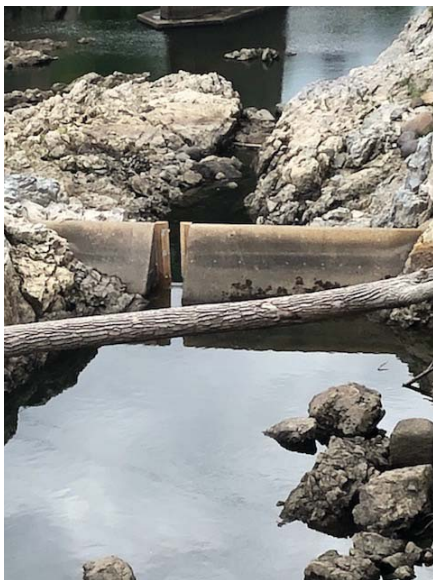
PHOTO 1 TEMPORARY BROAD-CRESTED WEIR (DEWATERED POST CONSTRUCTION)
