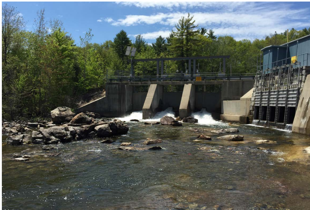
Canal Waste Gates from left abutment
