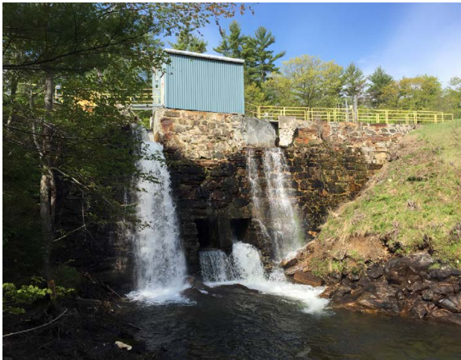
West forebay sluice discharge to lower bypass at powerhouse
