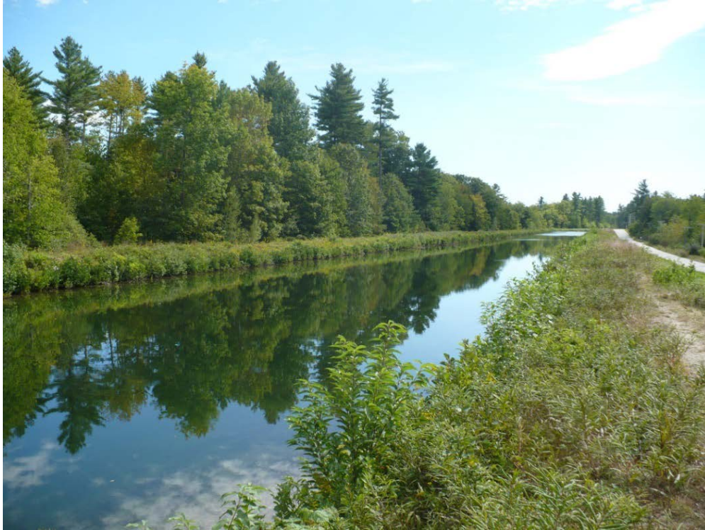
Canal looking downstream
