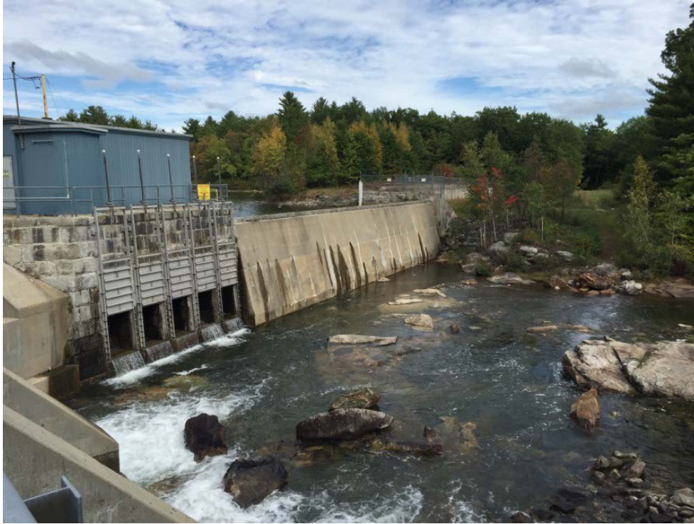
Spillway and Rivergate structure, (Bypass Reach)
