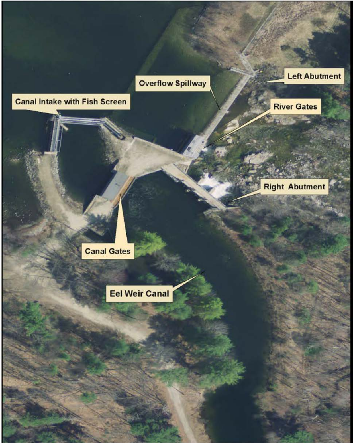
Fig. 3 – Close-up of Project Features
